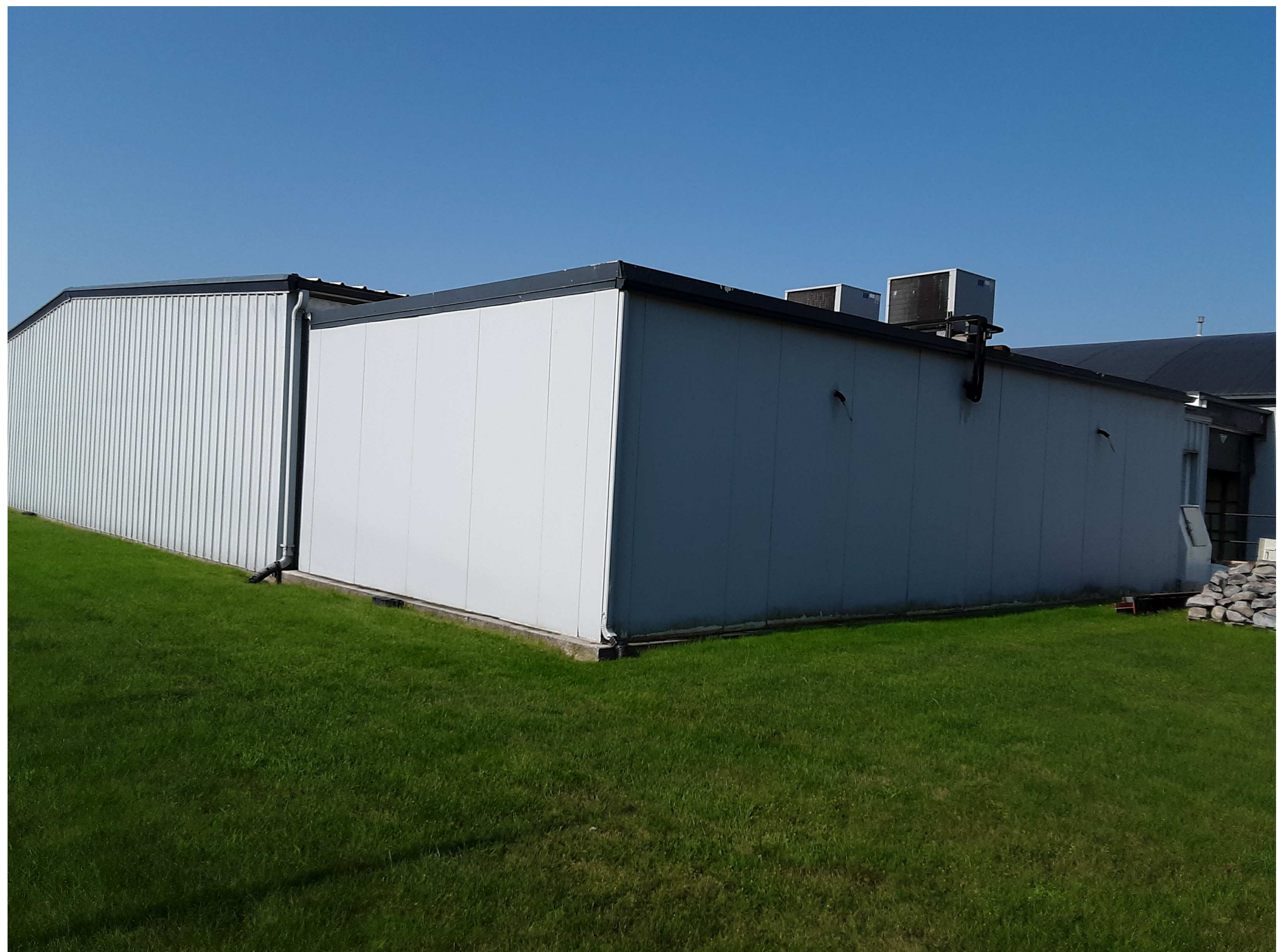
NORTHEAST CORNER OF EXISTING COOLER
