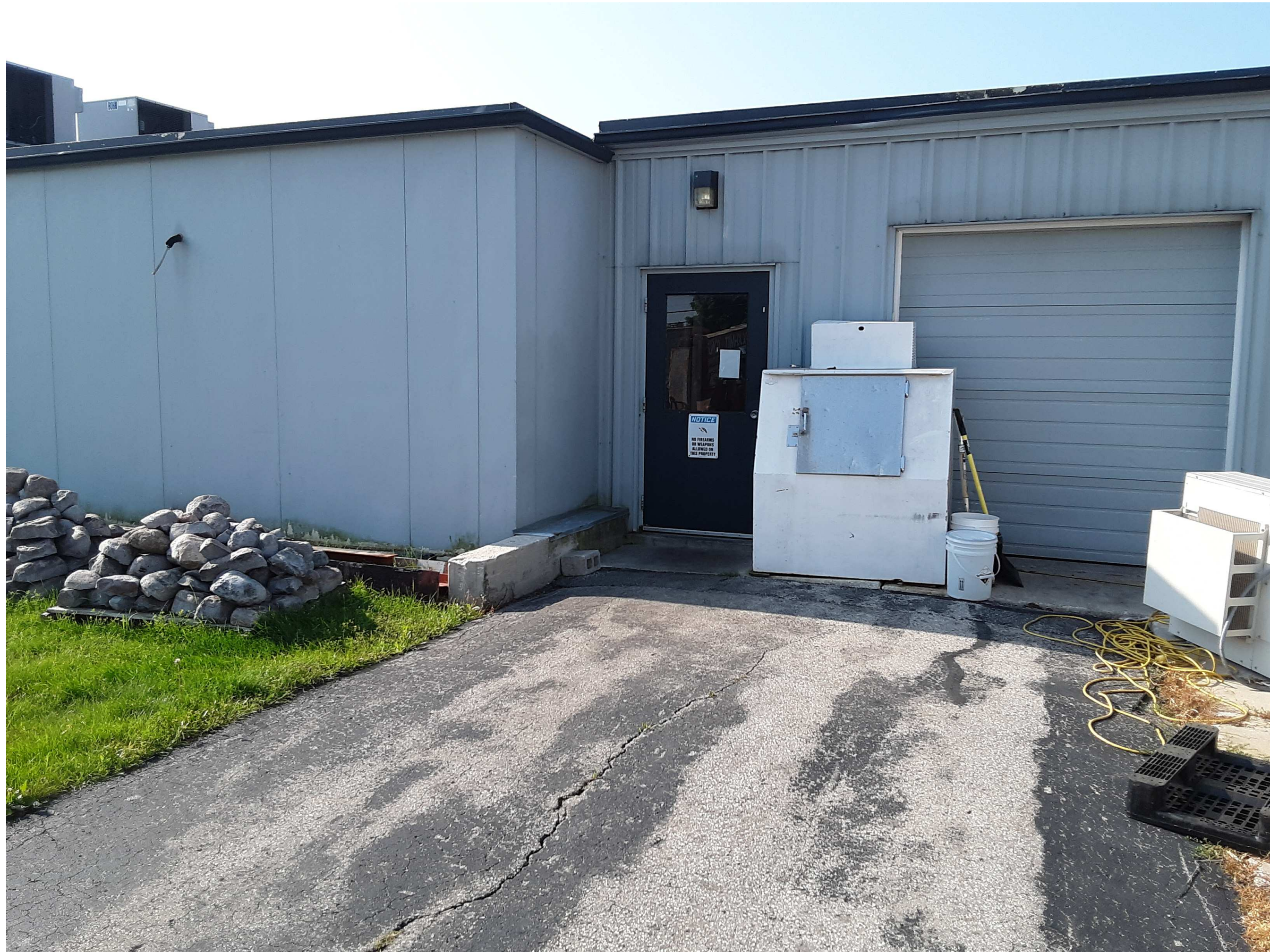
NORTH ELEVATION AT EXISTING GRADE-LEVEL LOADING DOCK
