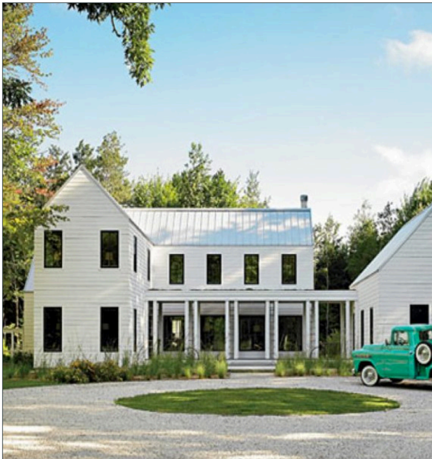
The simple repetition of windows and porch columns creates a rhythm
