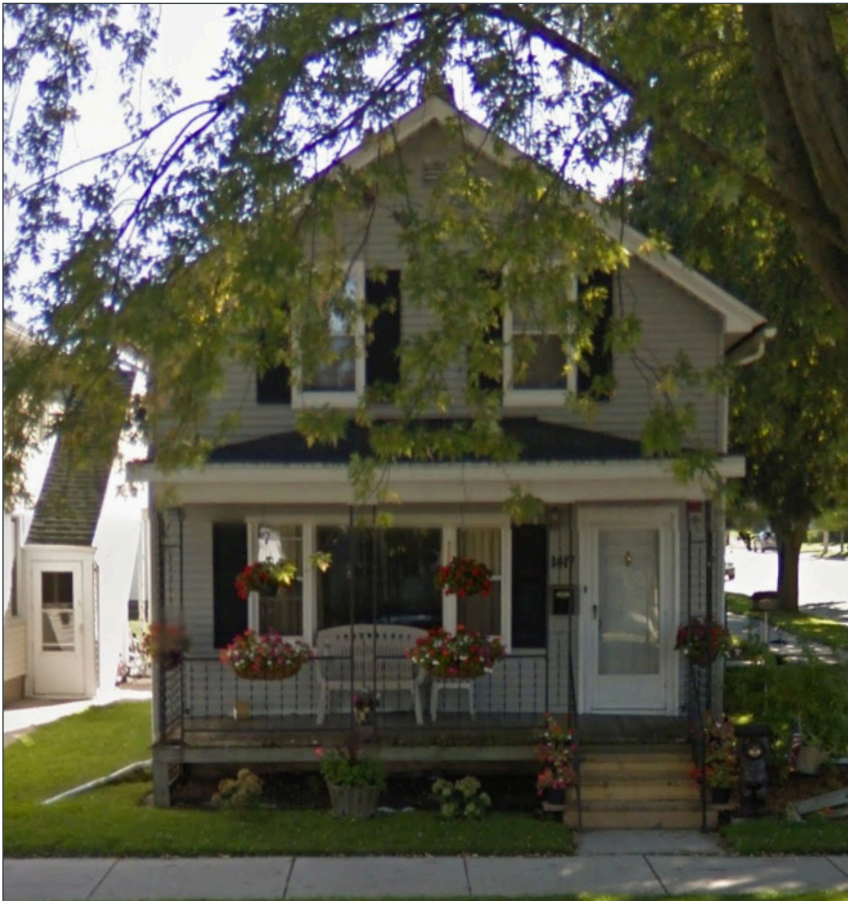
Modest size, lap siding, symmetrical window arrangement & steeply pitched roof. (Wisconsin Ave).
