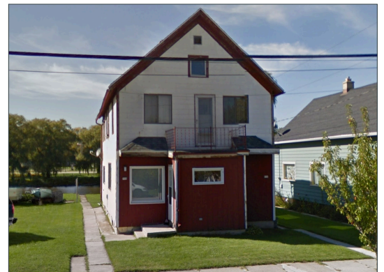
A two story home with a steeply pitched roof. (15th St)
