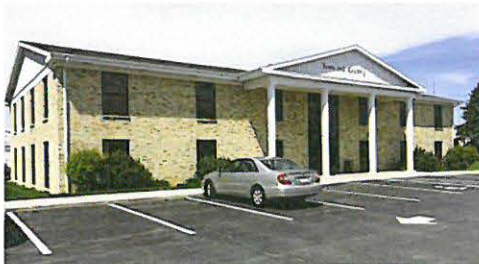
2108 Kohler Memorial Drive
