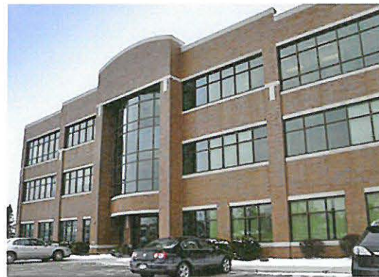
2124 Kohler Memorial Drive
