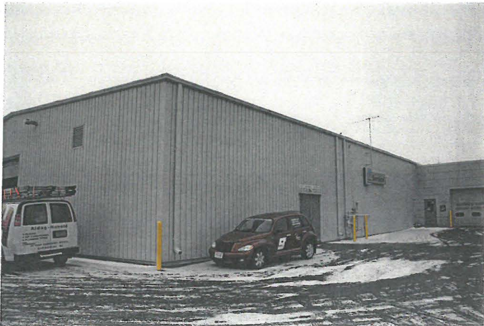
NORTHEAST CORNER OF SERVICE BAY...LOOKING SOUTHWEST
