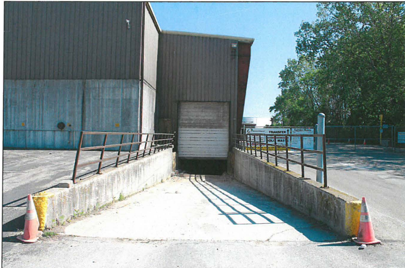
VIEW OF WEST PIT
