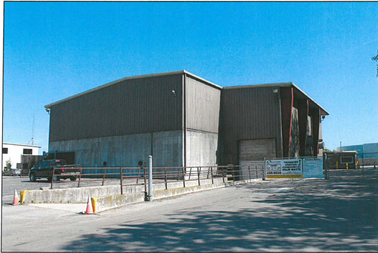
OVERALL VIEW AT NORTHWEST CORNER
