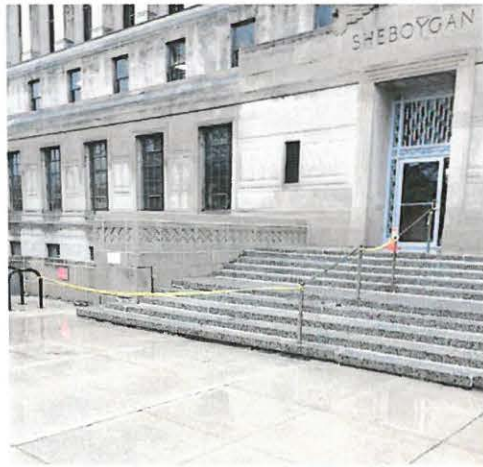
Stair & North Wall
