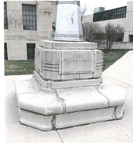
South Flagpole Base
