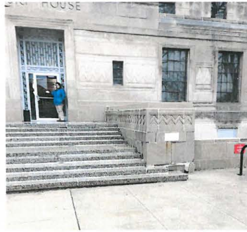
Stair & South Wall
