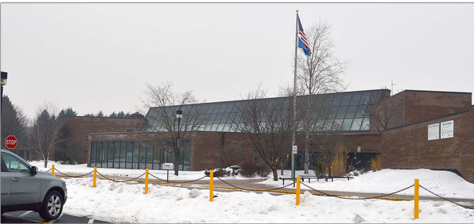
South Elevation - Main Entry
