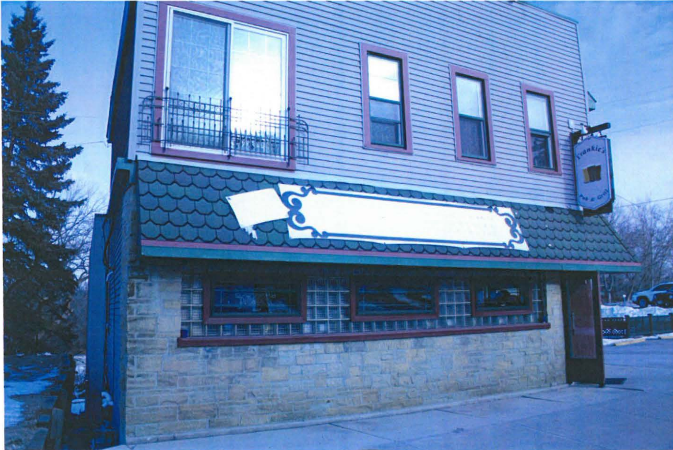
NEIGHBORING BUILDING TO THE EAST...LOOKING NORTH
