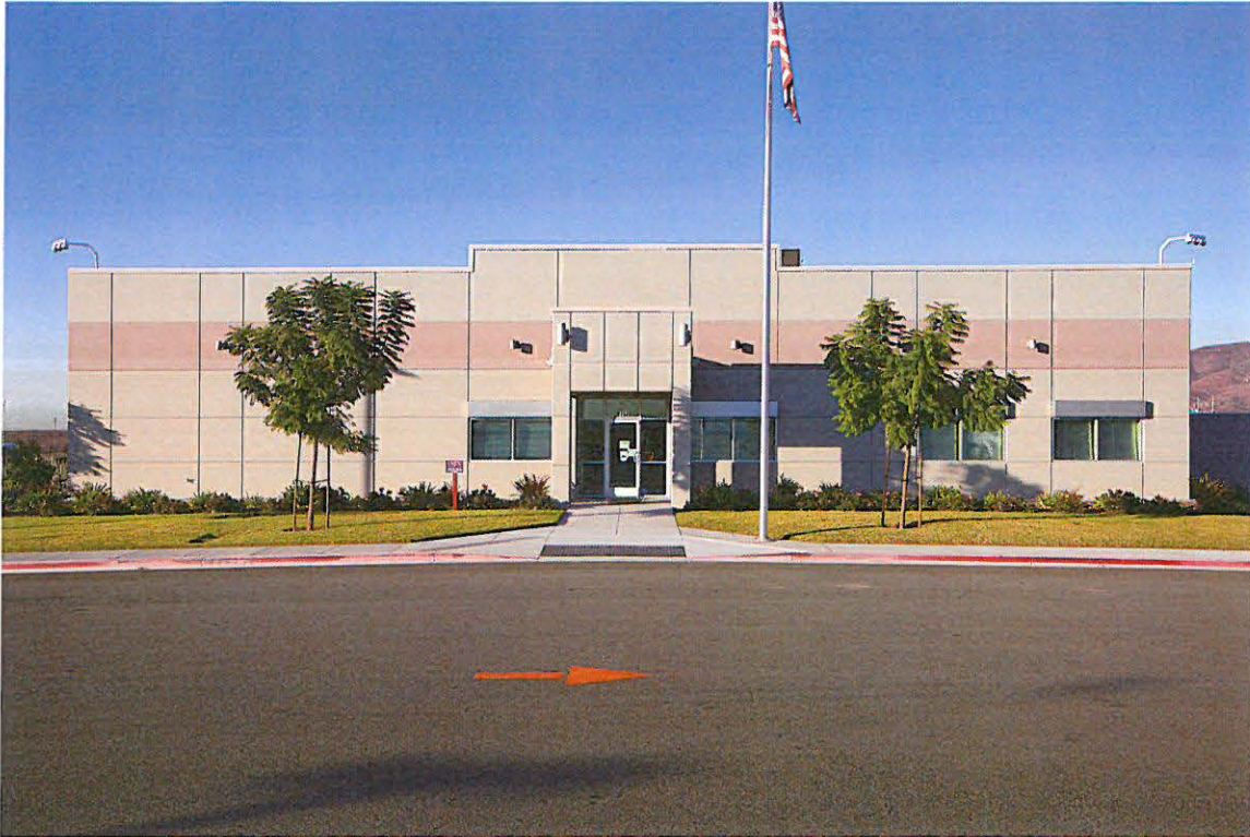
Picture of precast panel at main entrance
