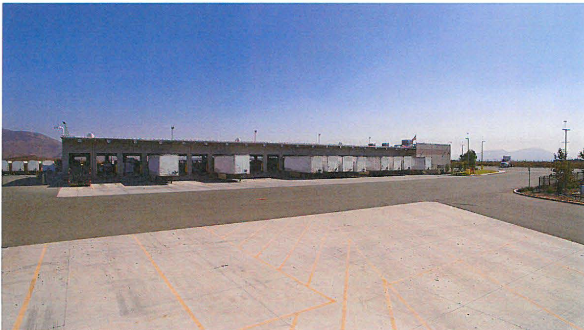
Picture of dock area and metal wall panels
