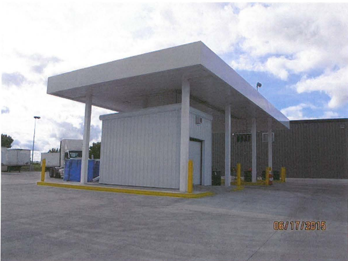
Picture of lube shed
