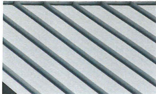
Standing Seam Metal Roof
