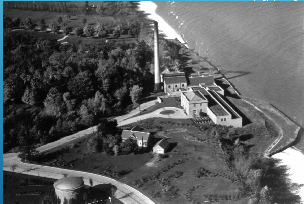
Water Utility plant and grounds circa 1935
