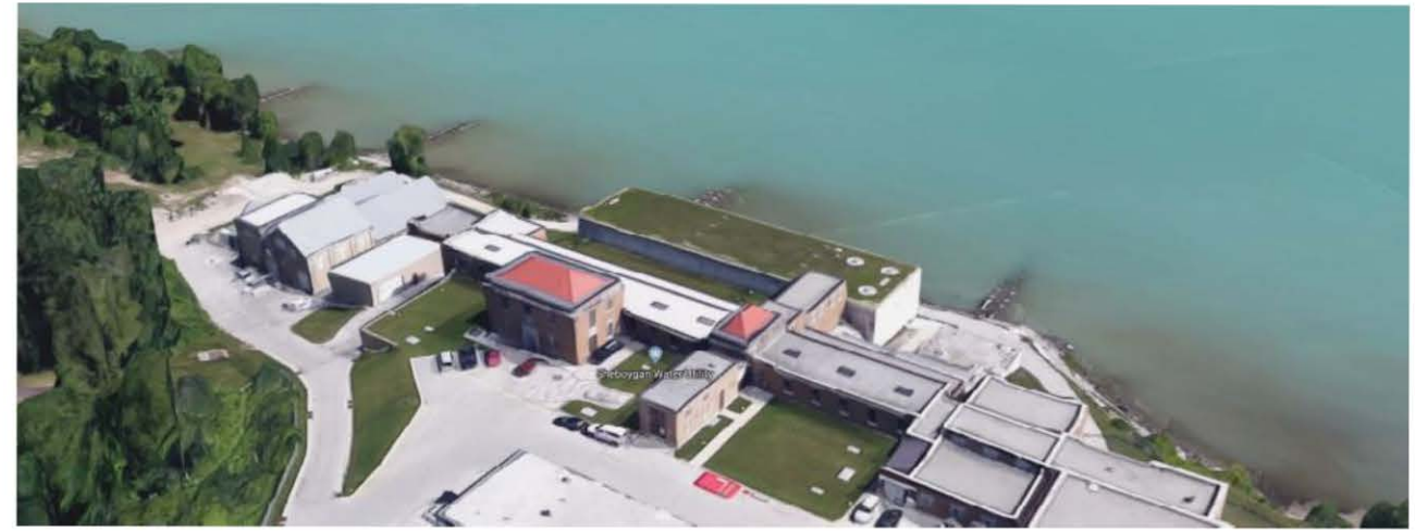
Aerial view of existing water plant
