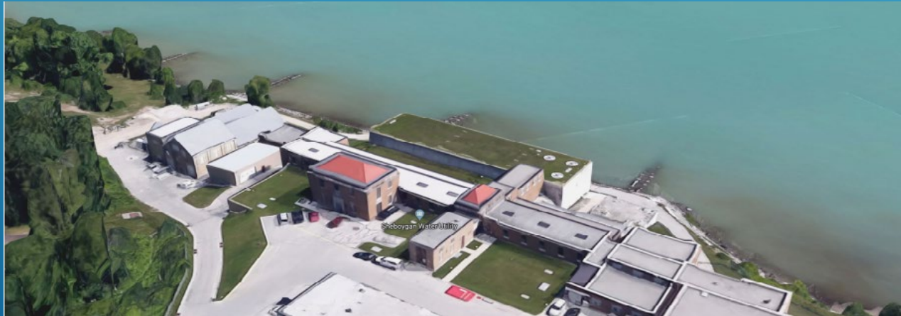
Water Utility plant and grounds 2020
