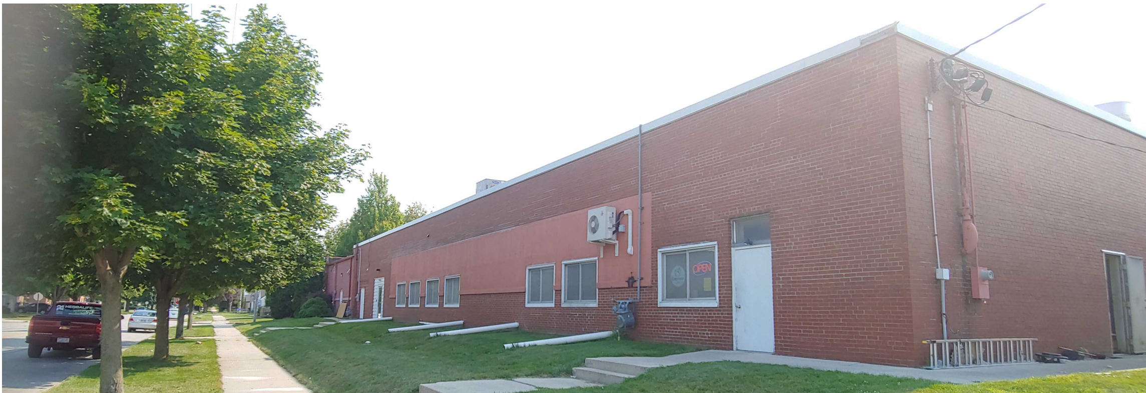
EXISTING CONDITIONS - EAST ELEVATION (NORTH END)
