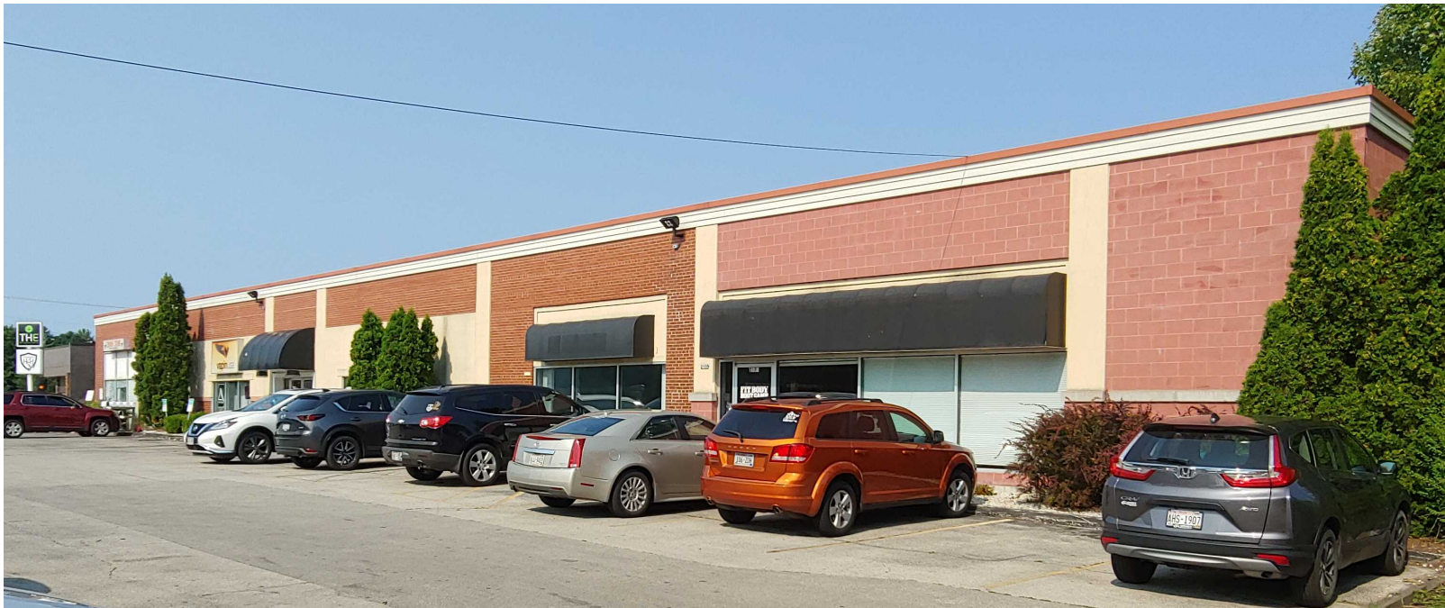
EXISTING CONDITIONS - WEST ELEVATION (SOUTH END)
