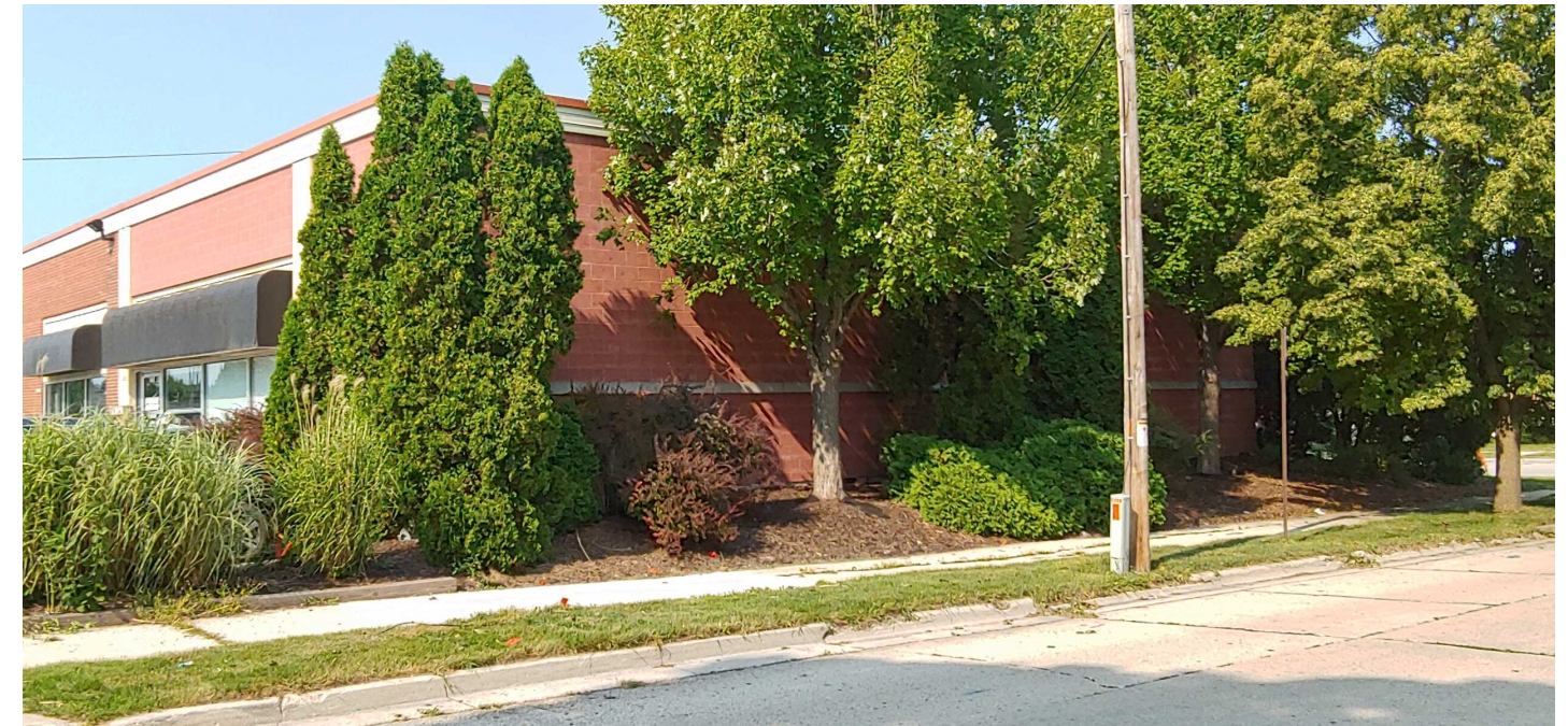
EXISTING CONDITIONS - SOUTH ELEVATION (WEST END)
