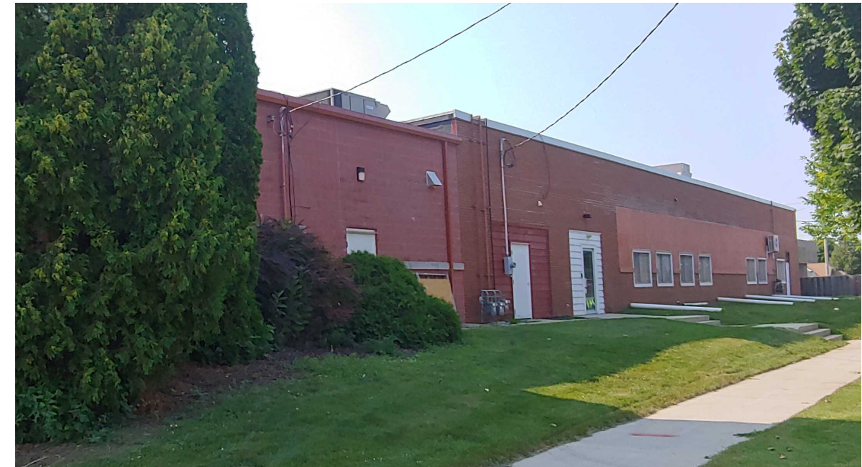
EXISTING CONDITIONS - EAST ELEVATION (SOUTH END)
