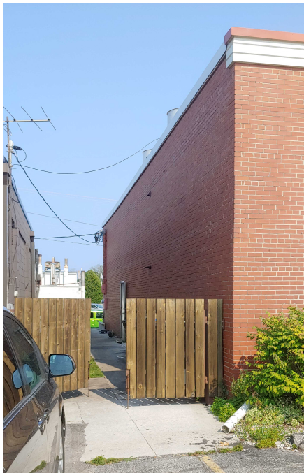
EXISTING CONDITIONS - NORTH ELEVATION (WEST END)
