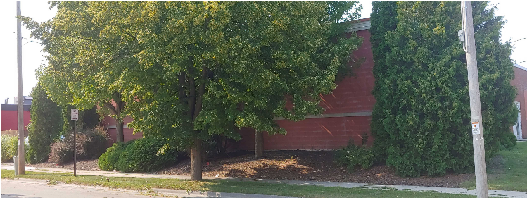
EXISTING CONDITIONS - SOUTH ELEVATION (EAST END)
