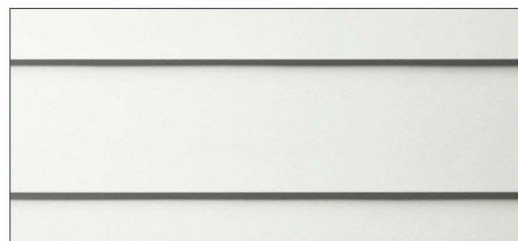
Painted Clapboard Siding and Trim
