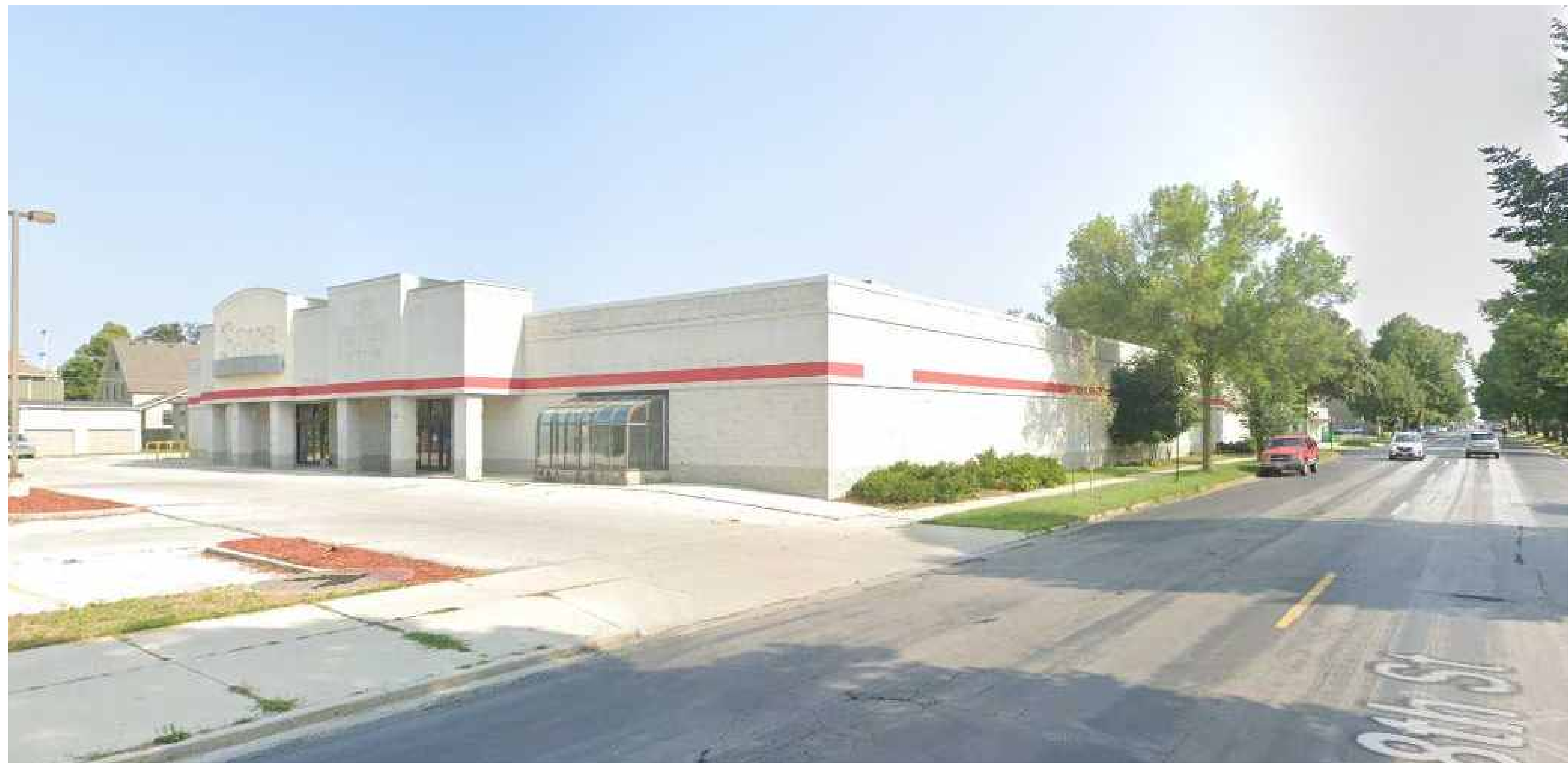
EXISTING BUILDING VIEW FROM NORTHWEST - 8TH STREET
