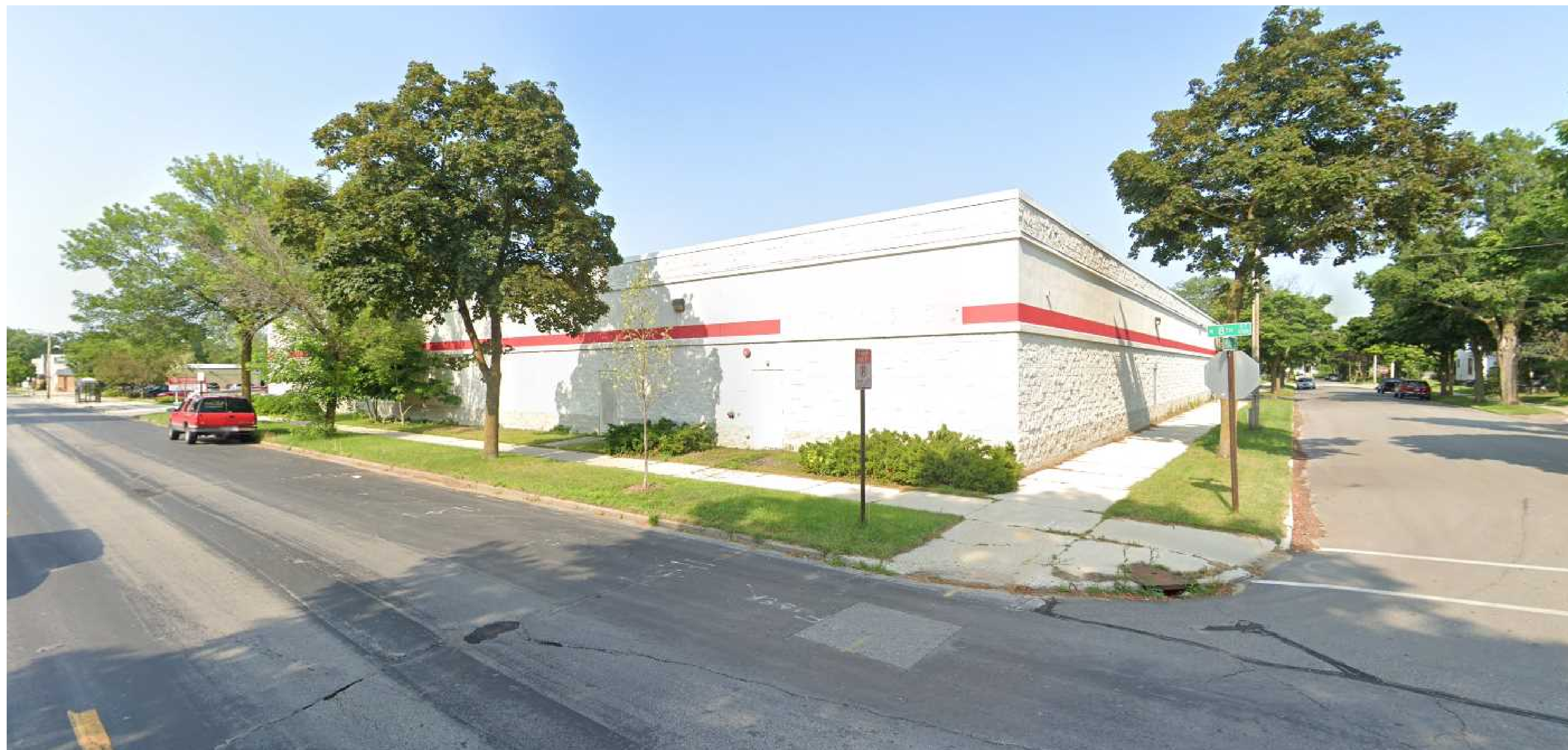
EXISTING BUILDING VIEW FROM SOUTHWEST - 8TH STREET & ZIMBAL AVE.
