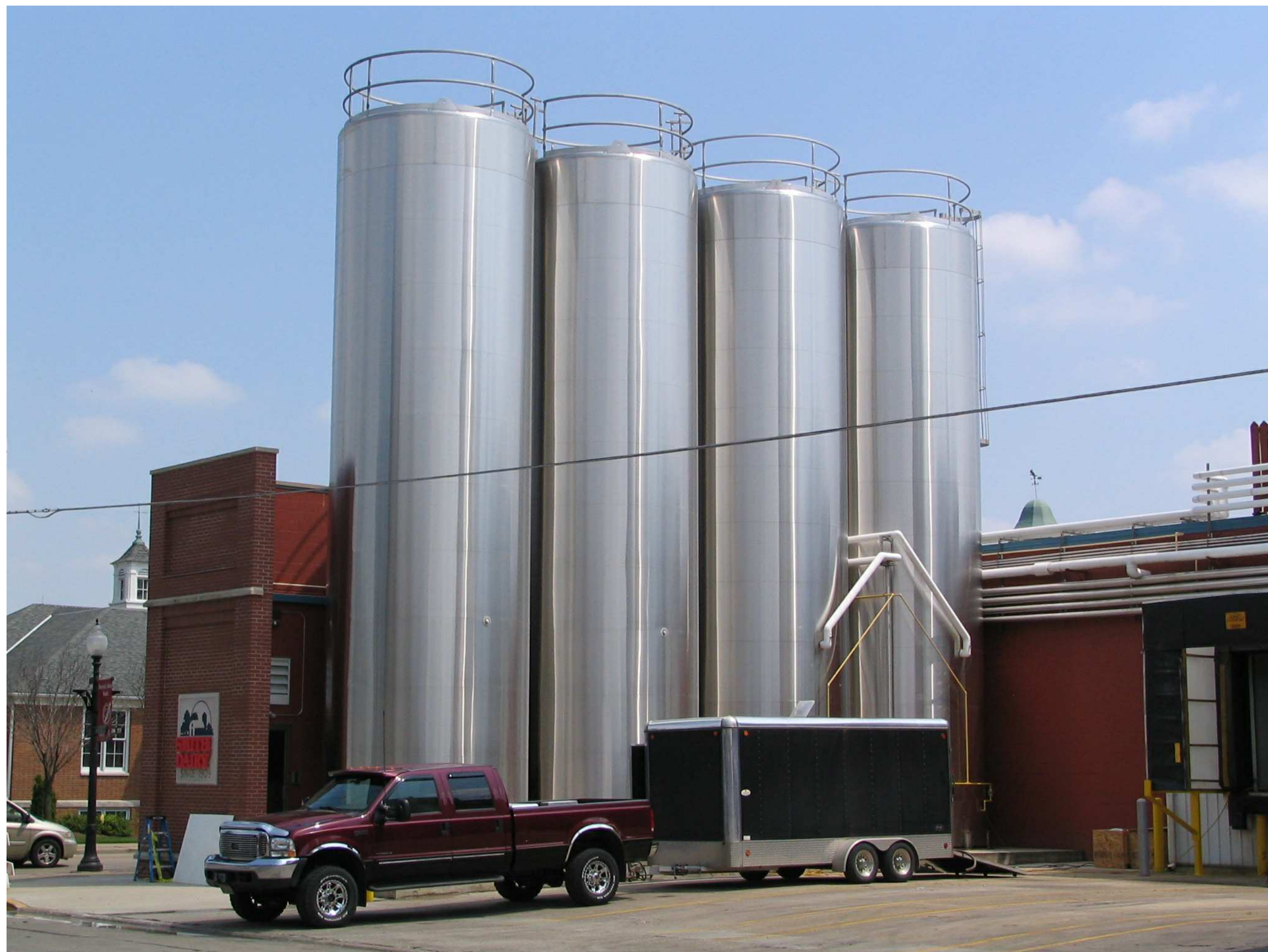
BUILDING WITH TANKS SIMILAR TO PROPOSED PROJECT
