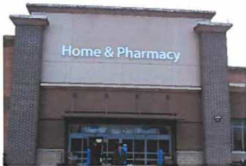
Existing 2'-6" Home & Pharmacy sign Will be replaced with a new 2'-6" Home & Pharmacy sign.
