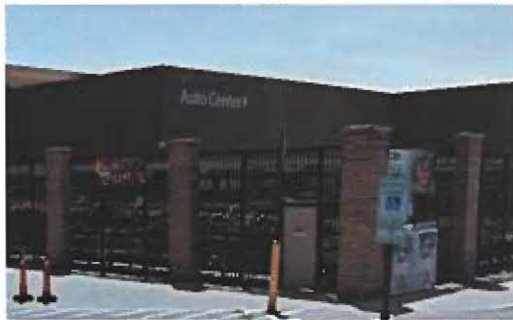
Existing 2'-0" Auto Center sign with right arrow Will be replaced with new 2'-0" Auto Center sign with arrow.
