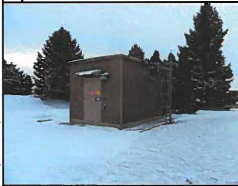
C EXISTING EQUIPMENT SHELTER
