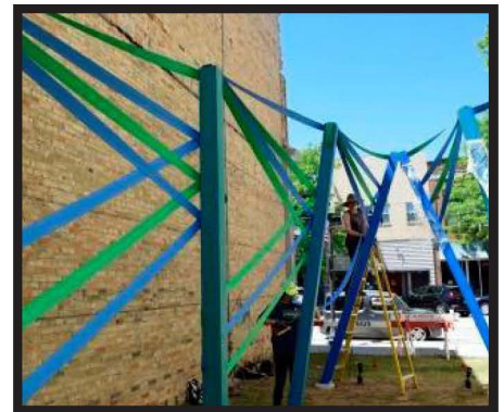
Installation of "Opening (Walk Through #1)" by Diana Gabriel. Photo credit: City of Sheboygan.
