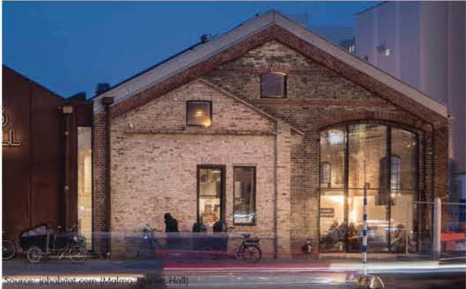
▲ (Middle image) Existing structure at the corner of Pennsylvania Avenue and N. Commerce Street. (Bottom image) Adaptive reuse project example into restaurant, coffee shop, or other retail space.
