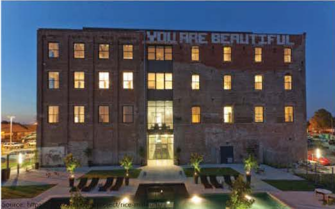
▲ (Middle image) Existing warehouse building along N. Commerce Street. (Bottom image) Adaptive reuse project example into residential lofts.
