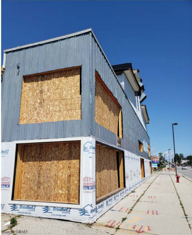
▲ A view of the rehabilitation of 822 N. 14th Street into a commercial space.
