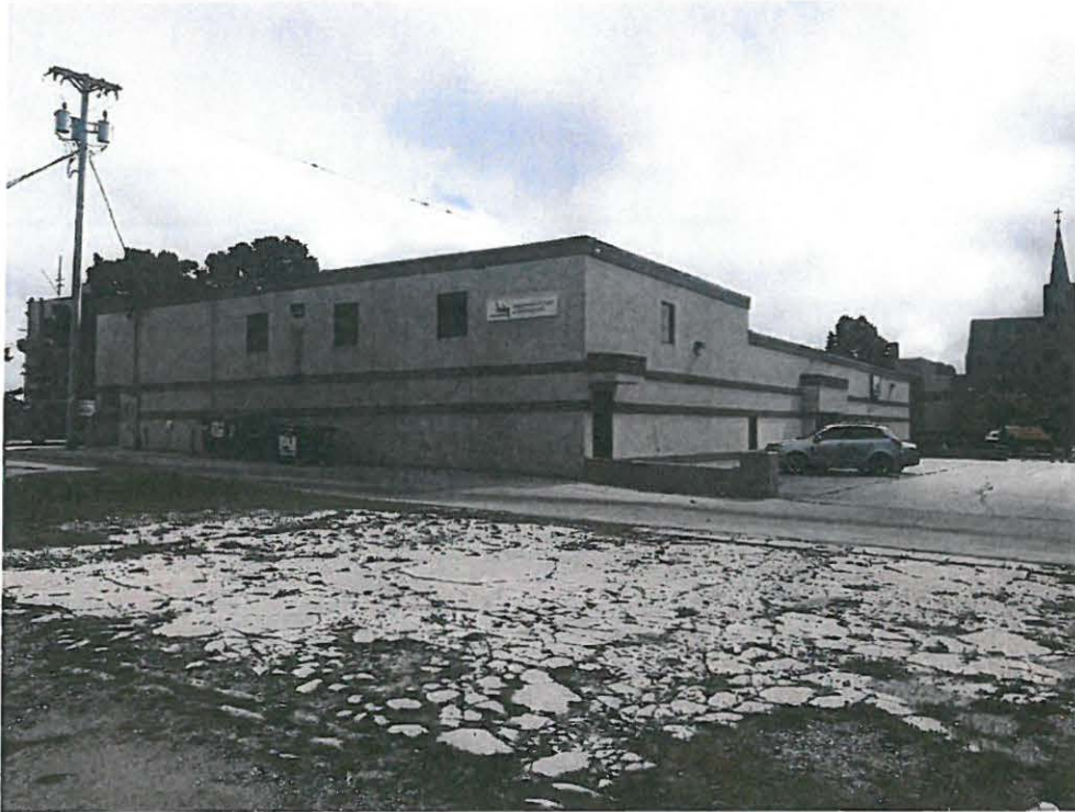
View of north side of building.
