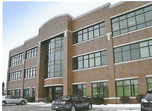
2124 Kohler Memorial Drive
