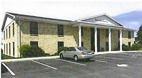
2108 Kohler Memorial Drive
