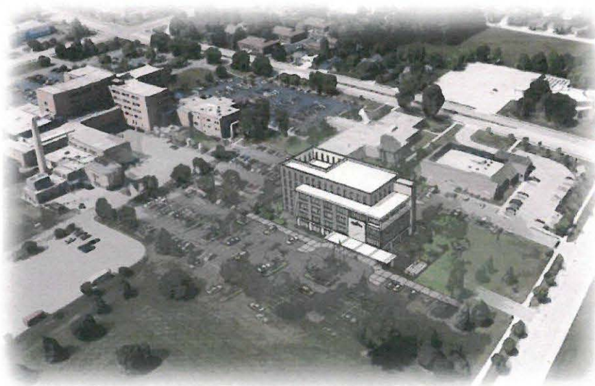
Bird's Eye View of location on St. Nick's Campus
