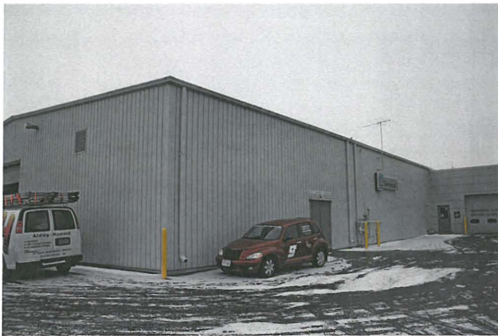
NORTHEAST CORNER OF SERVICE BAY...LOOKING SOUTHWEST
