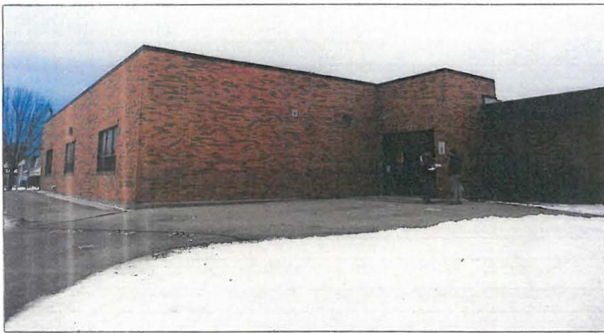
Northwest Classroom Elevation
