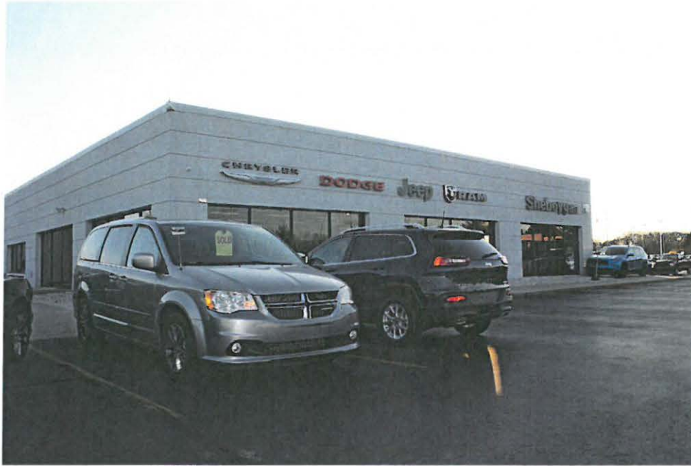
NORTHEAST ELEVATION OF SHOWROOM
