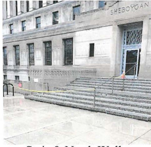
Stair & North Wall
