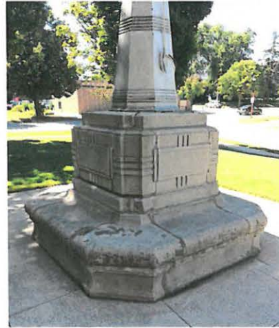
North Flagpole Base
