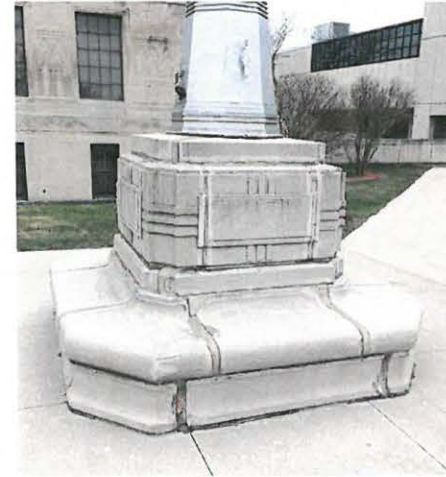
South Flagpole Base
