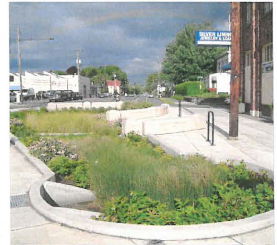
Green Infrastructure-rain garden
