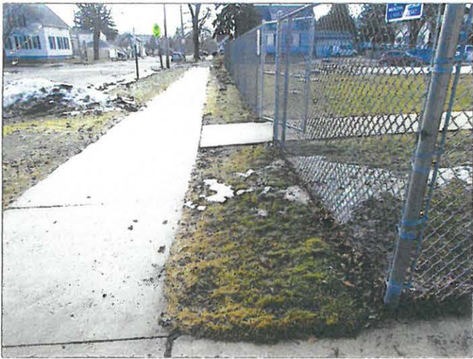
East end looking South
