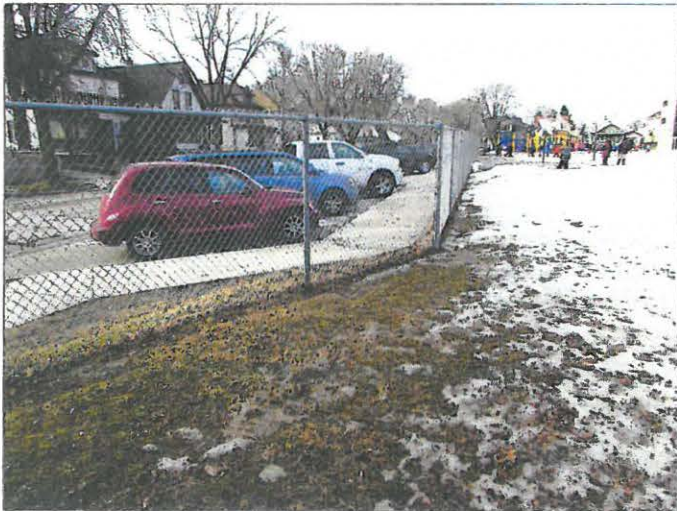
Southeast corner looking West
