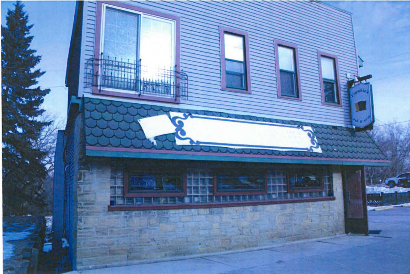
NEIGHBORING BUILDING TO THE EAST...LOOKING NORTH
