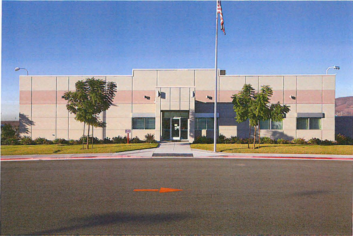
Picture of precast panel at main entrance
