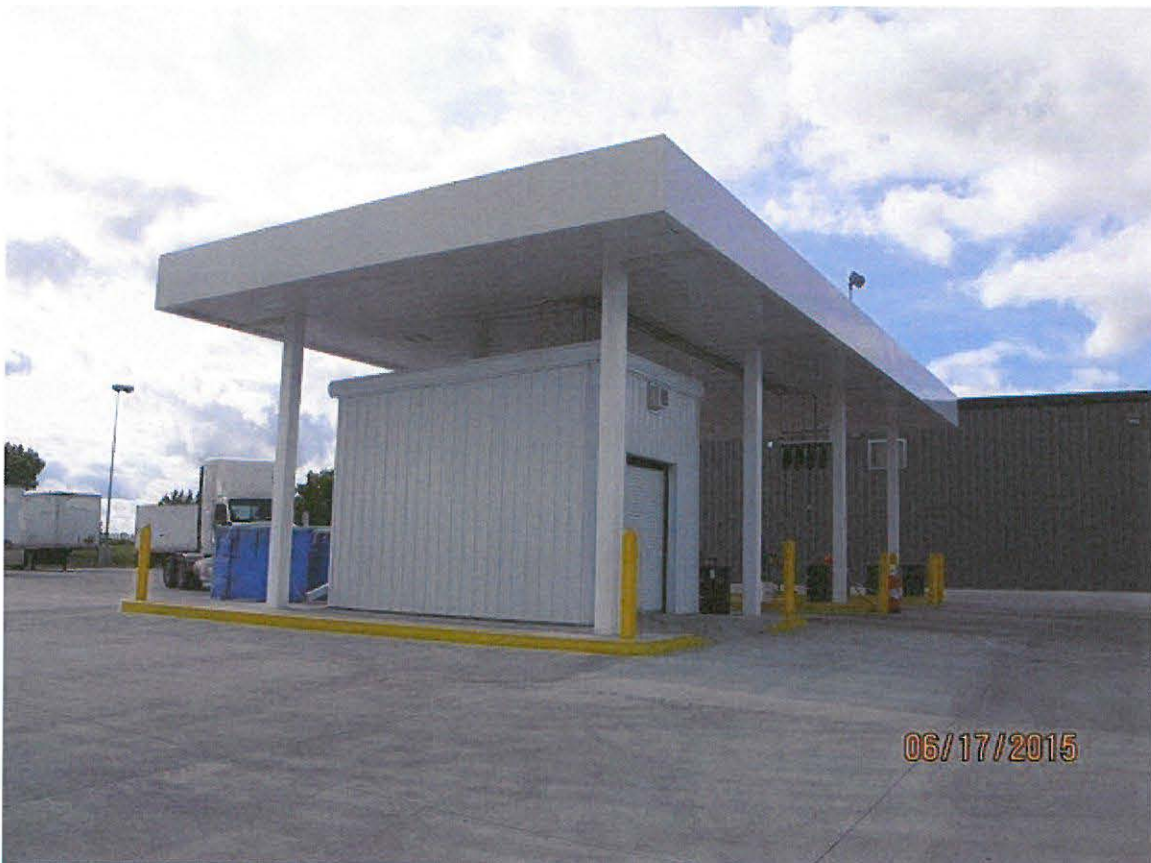
Picture of lube shed
