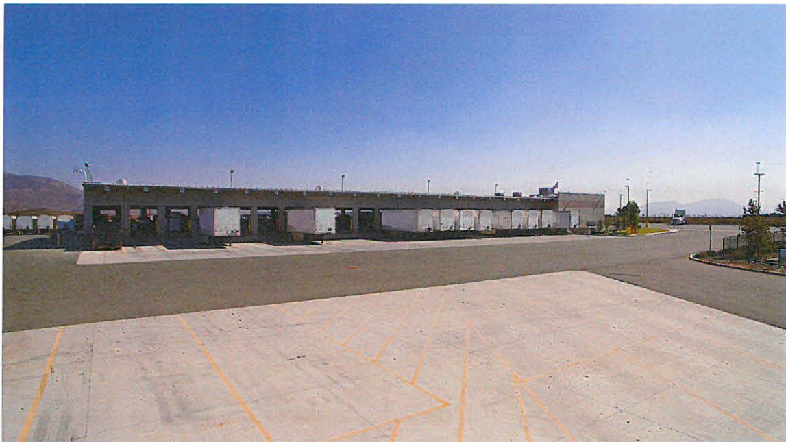
Picture of dock area and metal wall panels
