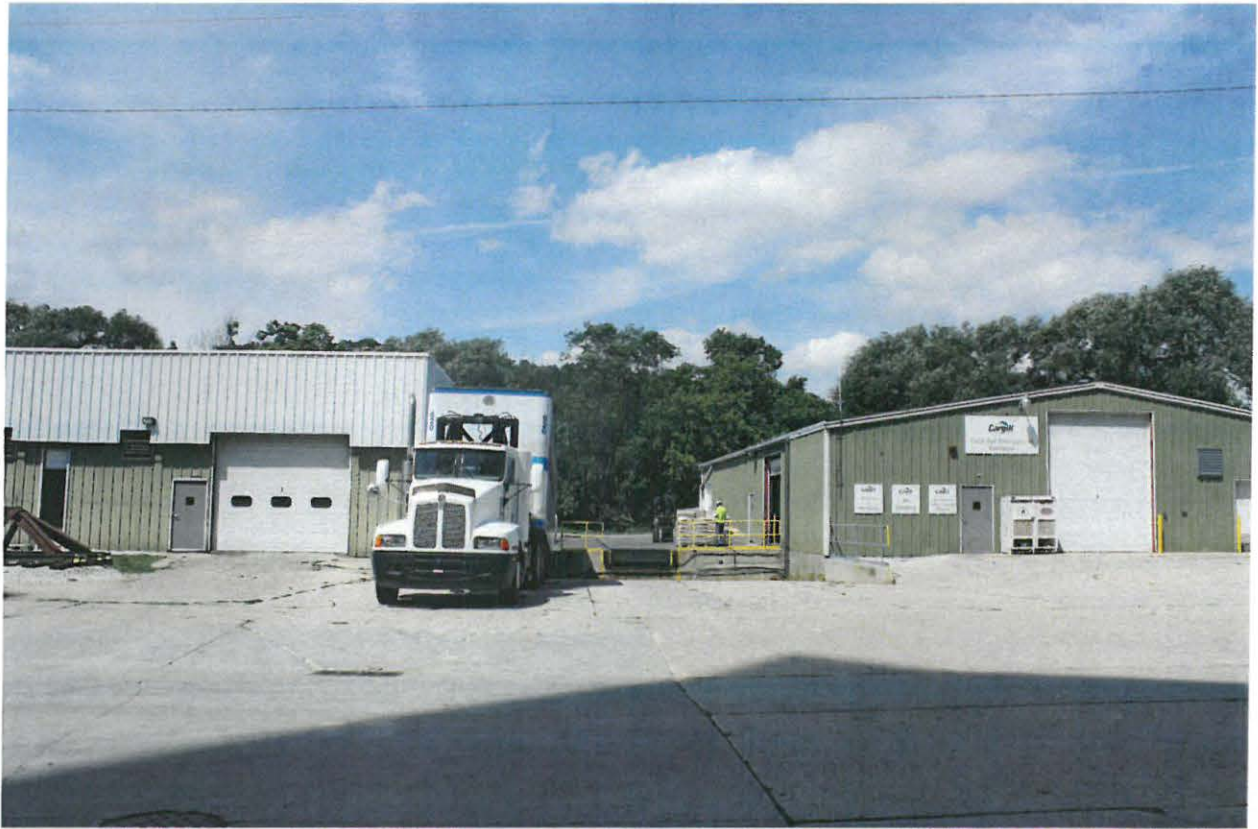
Looking Northwest at the project site
