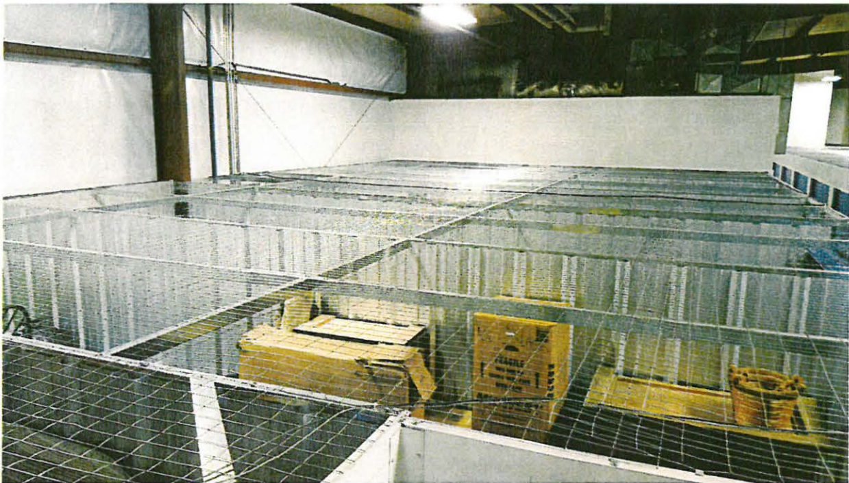
Picture of ceiling construction of inside units @ 3838 Enterprise Drive
