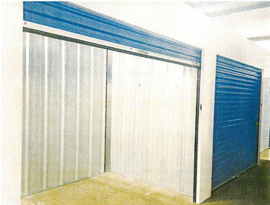
Inside view of a storage unit @ 3838 Enterprise Drive
