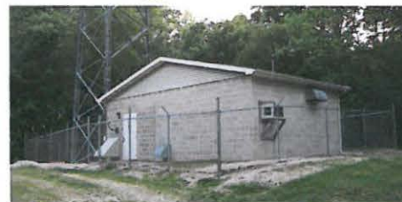
7 5 EXISTING TOWER SHED
