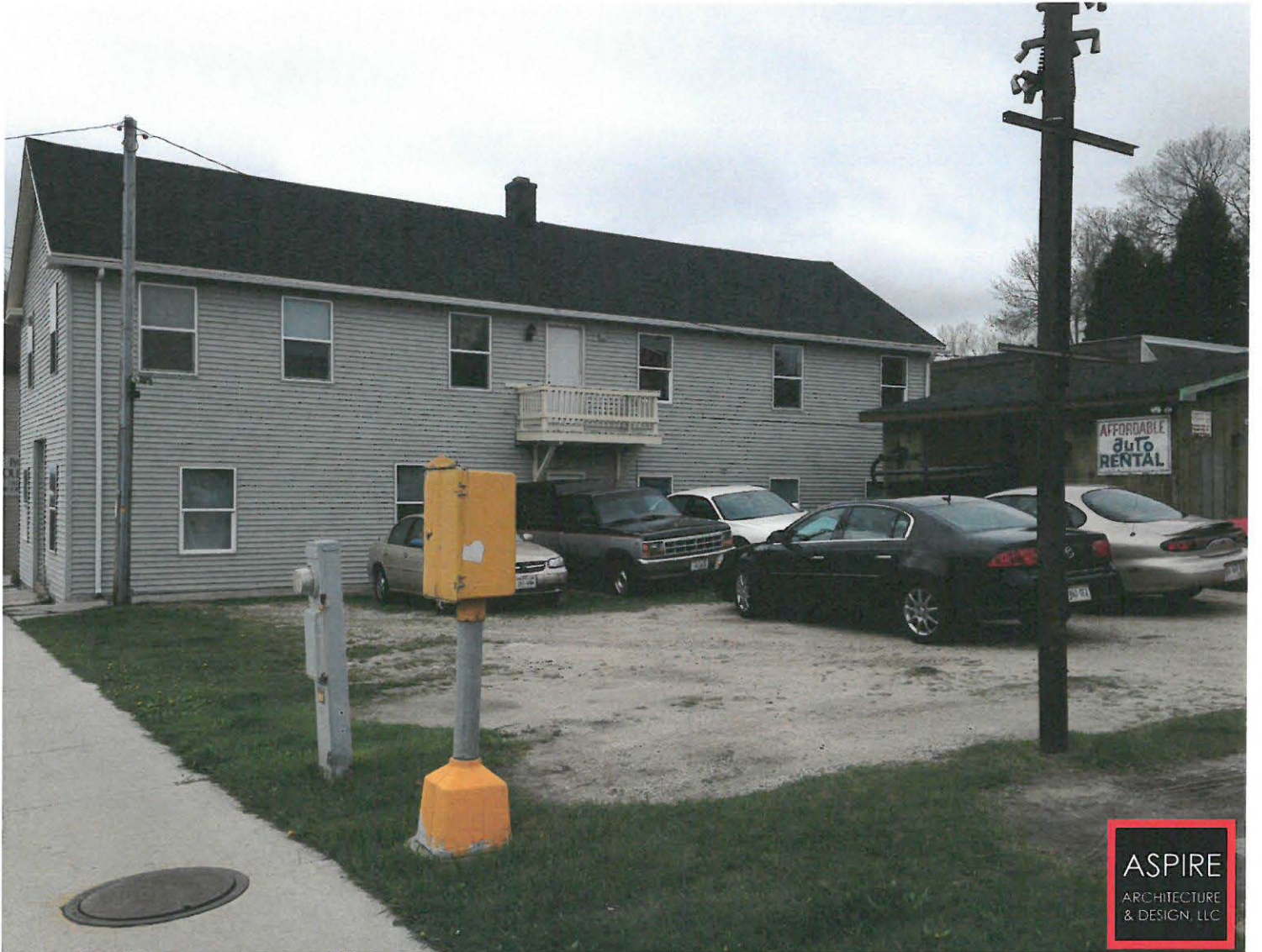
EXISTING PARKING LOT
