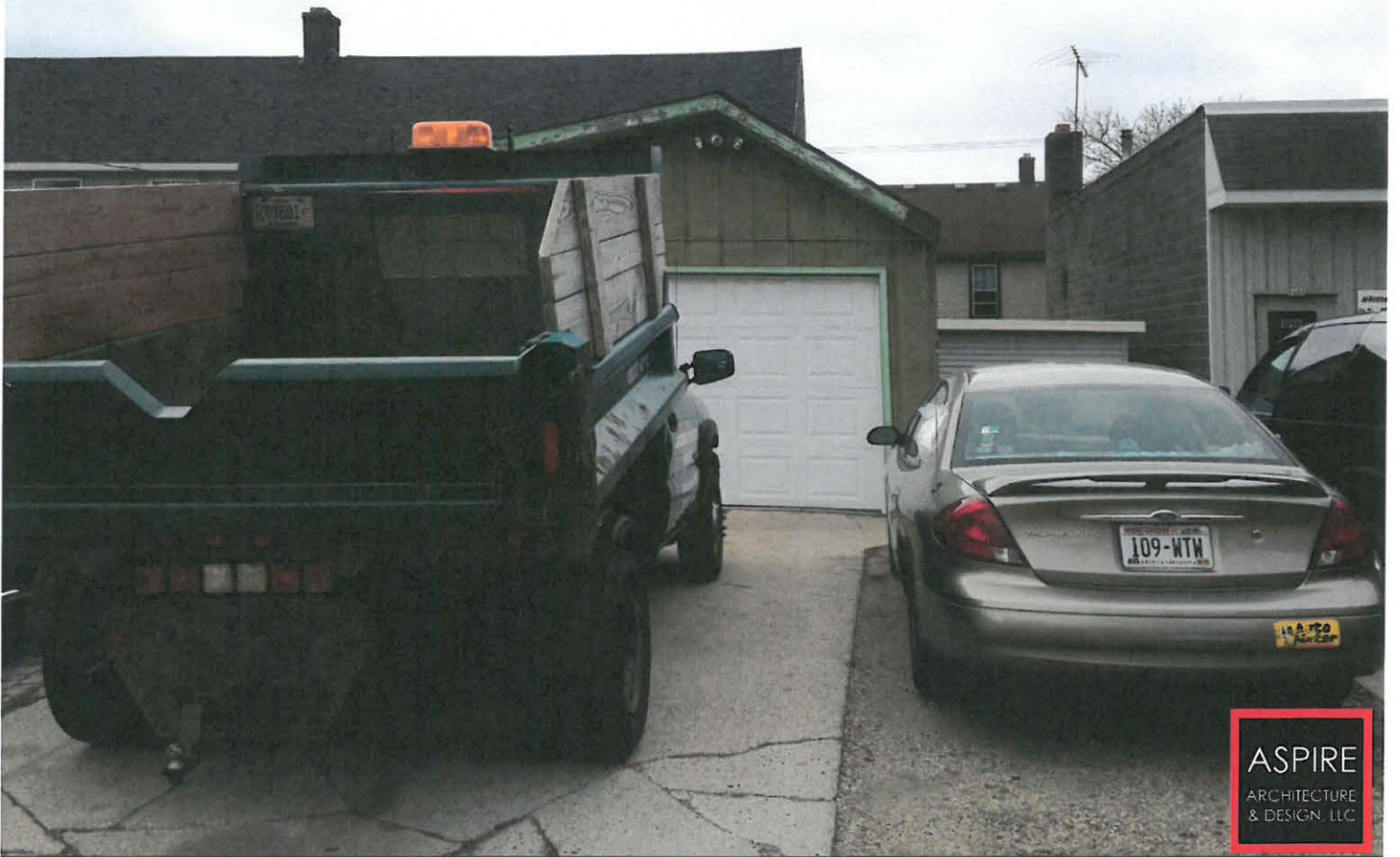
GARAGE TO BE RAZED
