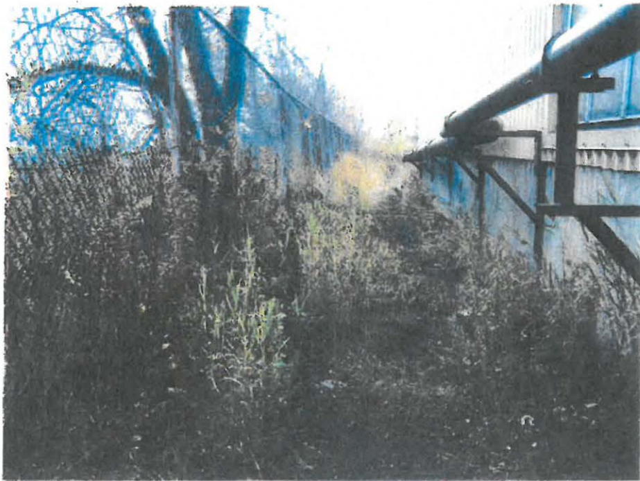
Photo 2: Looking south along the drainage swale in between the Crusher House (at right) and the fence along the top of the revetment.
