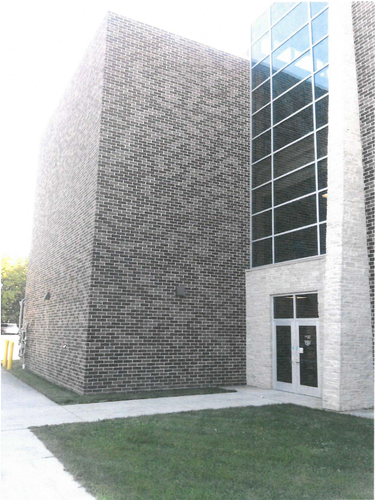
Existing North Entrance to Science Building
