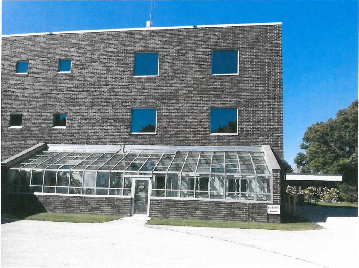
Existing West Façade
