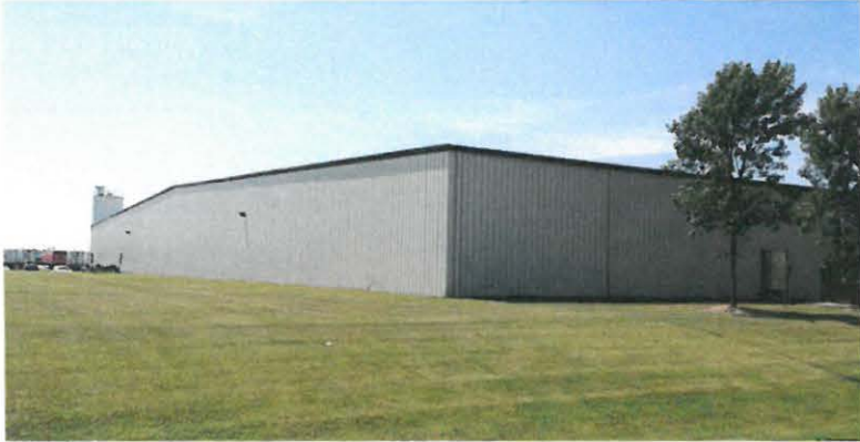
EXISTING VIEW - NORTHEAST CORNER OF TORGINOL FACILITY TAKEN FROM WEEDEN CREEK ROAD
