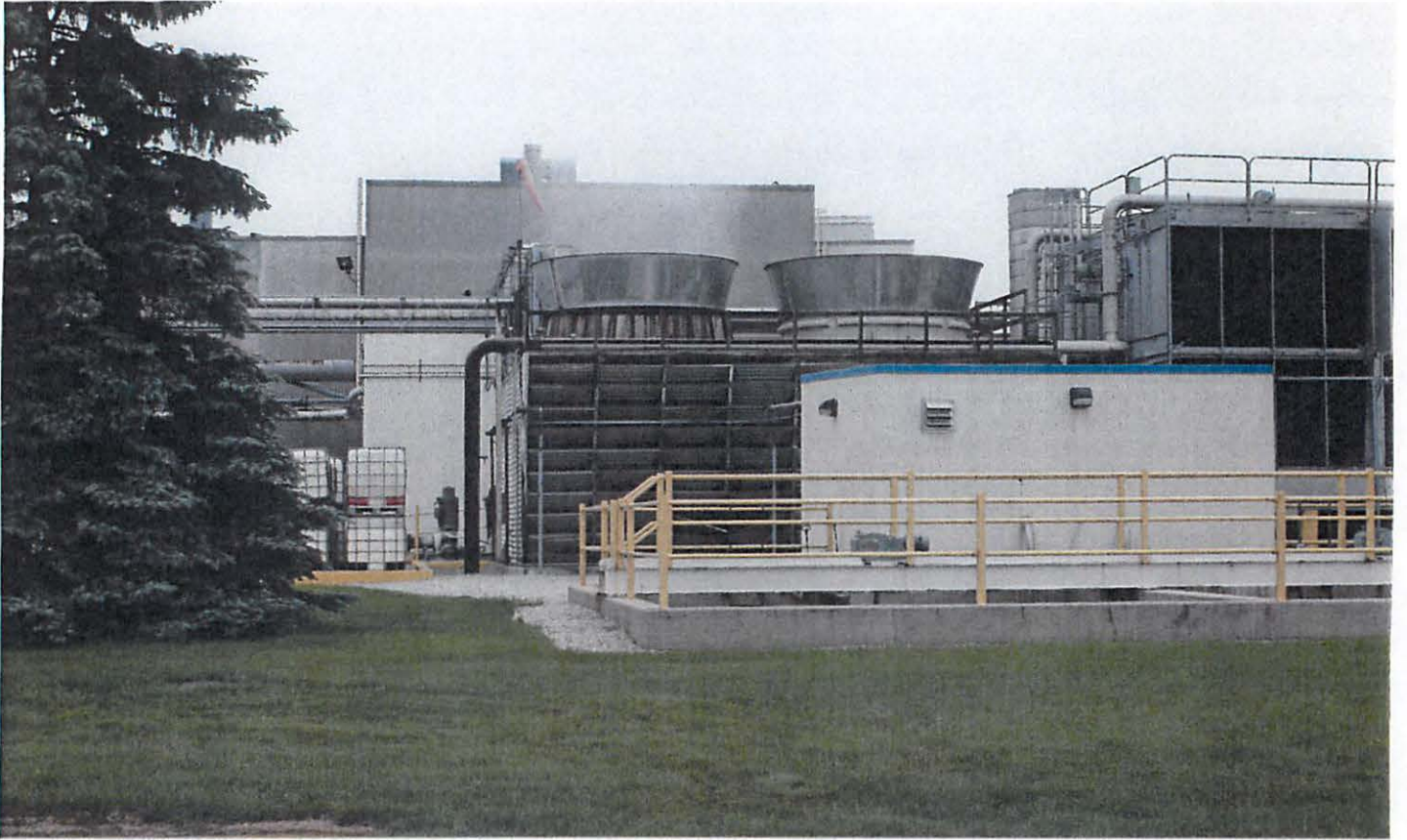
Looking West—Existing Pump House with Cooling Towers Beyond
