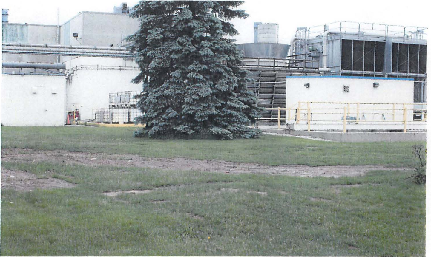
Looking Northwest—Site of New Cooling Tower, Existing Pump House Beyond
