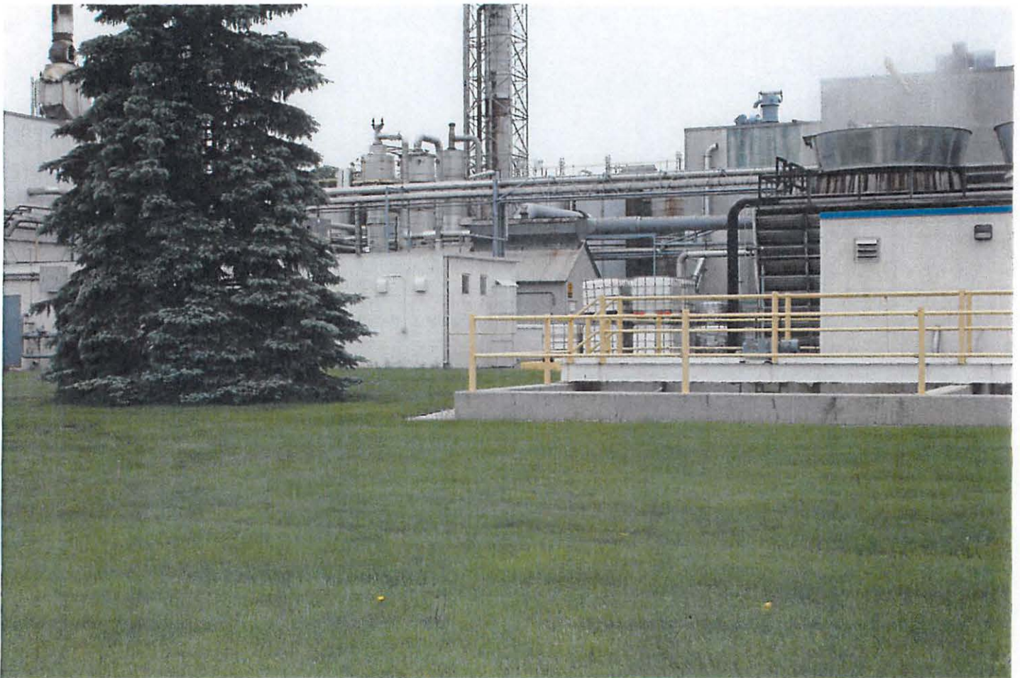
Looking Southwest—Site of New Cooling Tower, Existing Pump House at Right
