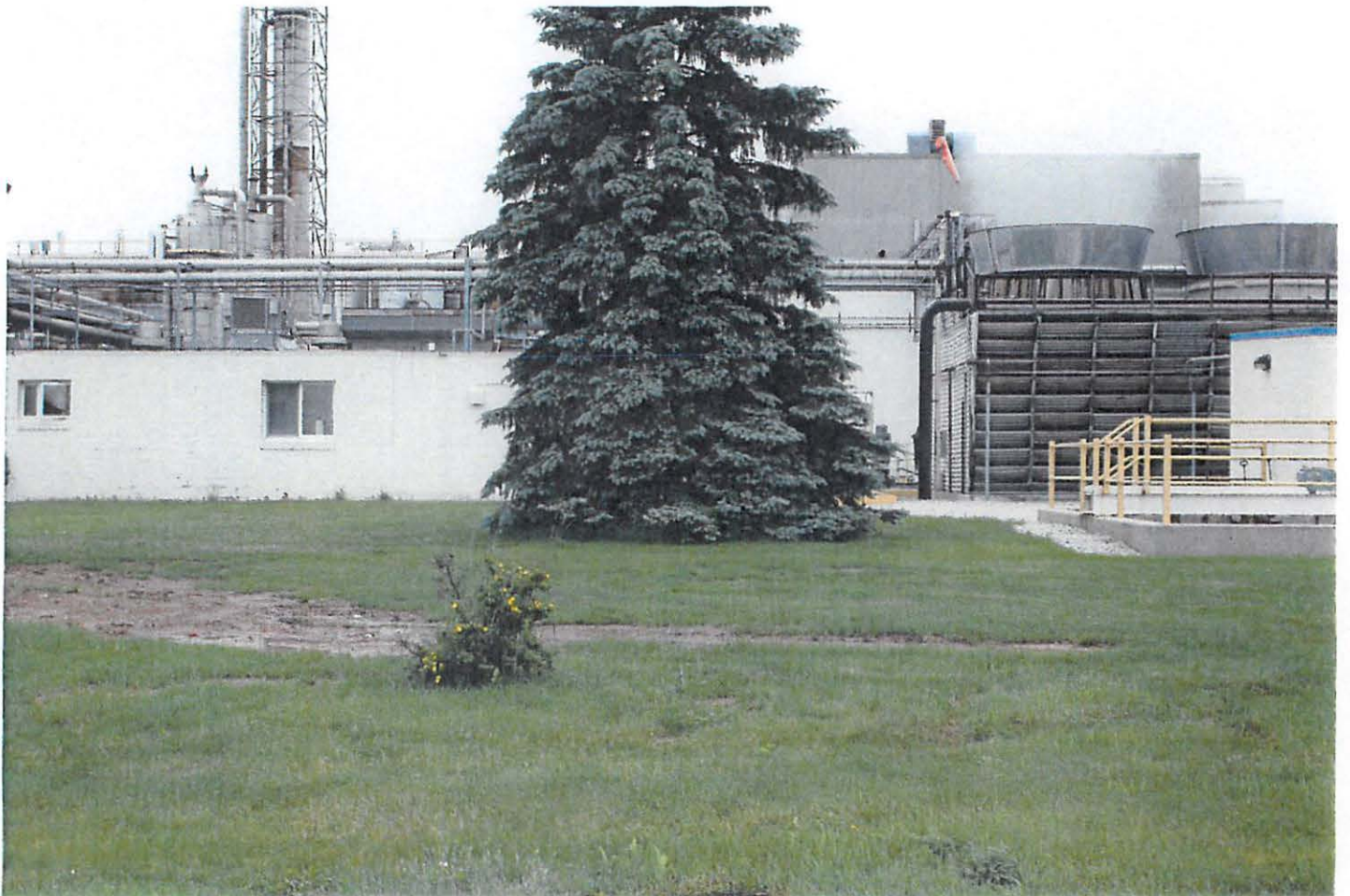
Looking West—Site For New Cooling Tower. Existing Cooling Tower at Right
