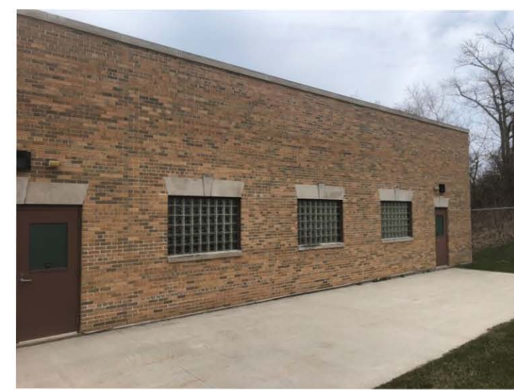
Typical existing materials
