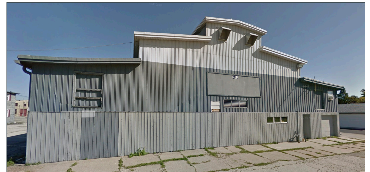
Original lumberyard across the street from proposed site (15th Street)
