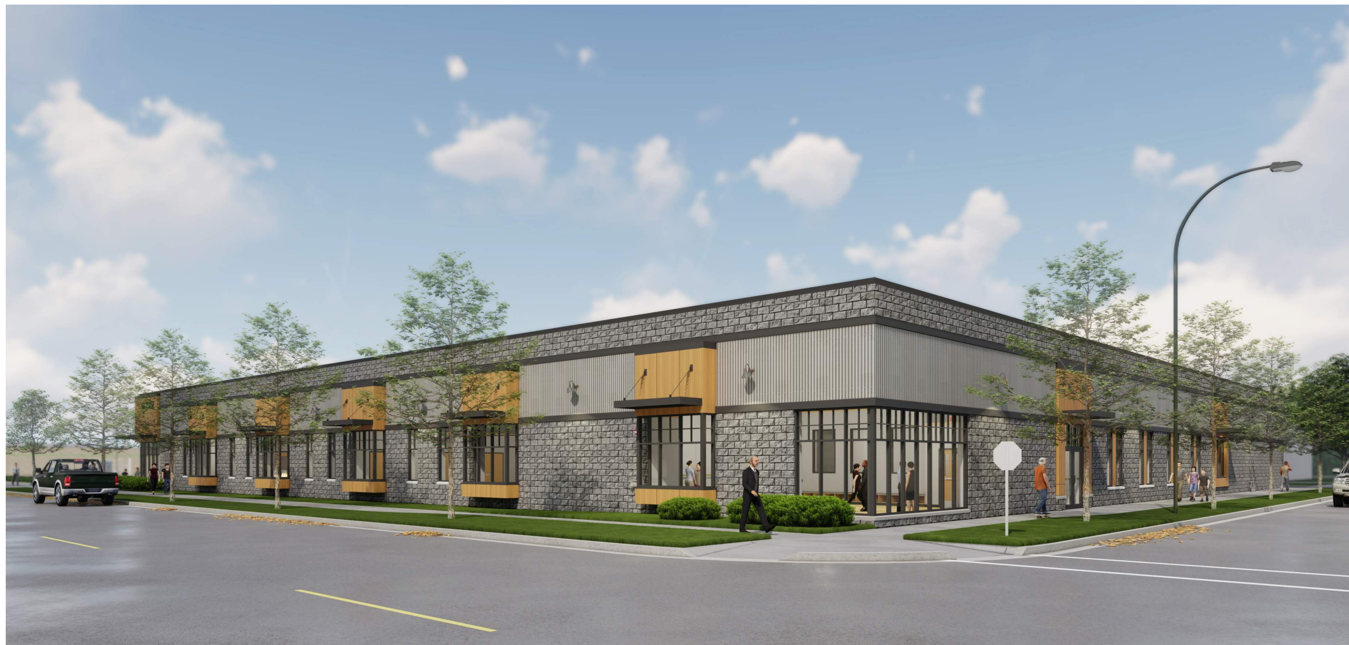
REMODELED BUILDING VIEW FROM SOUTHWEST - 8TH STREET & ZIMBAL AVE.
