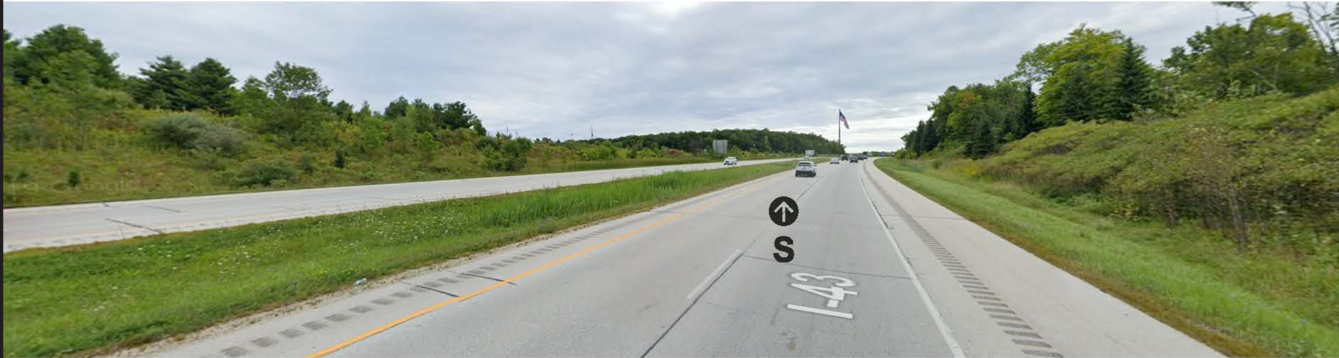
On Freeway - Southbound Lane - Looking South
