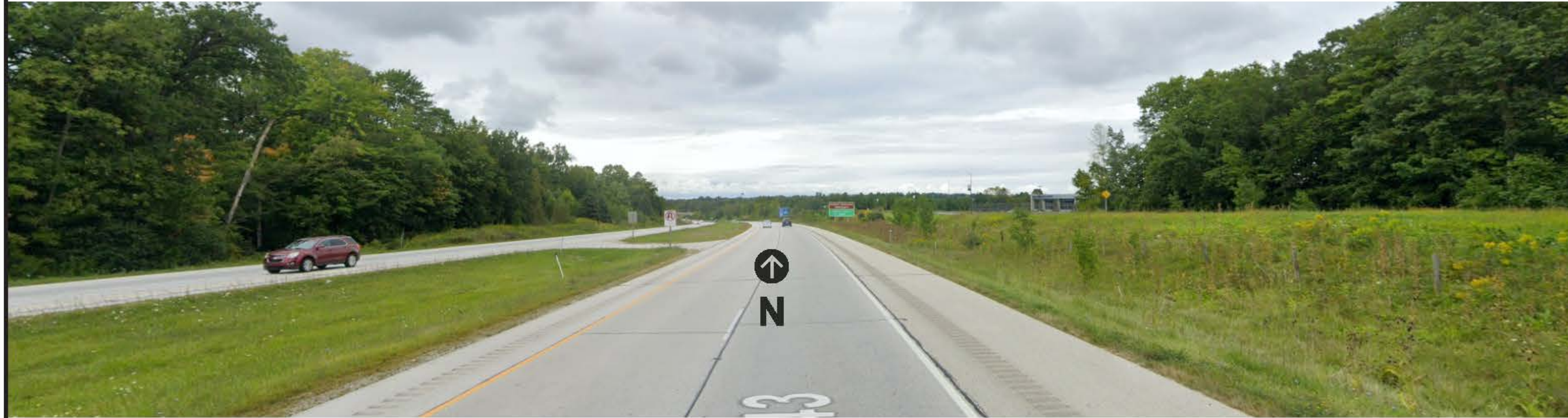
On Freeway - Northbound Lane - Looking North
