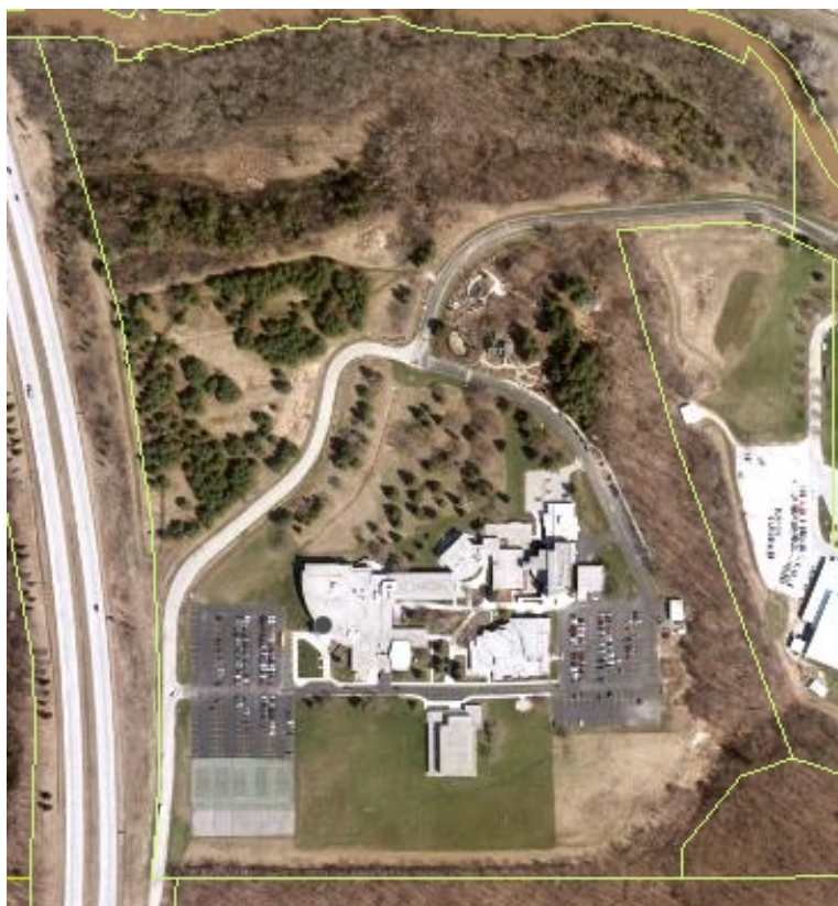
Overhead View Showing Property Lines in Yellow
