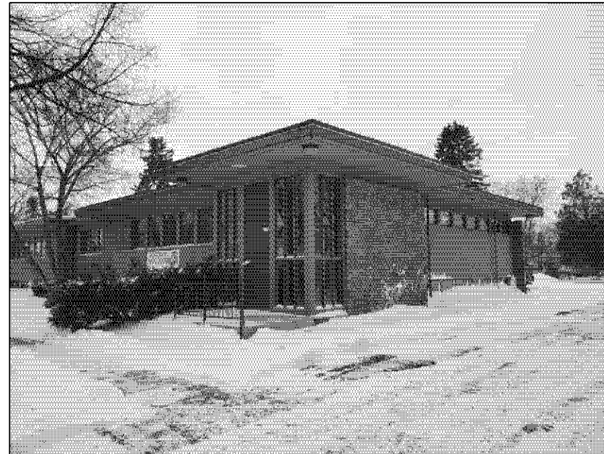
LOOKING SOUTH WEST
