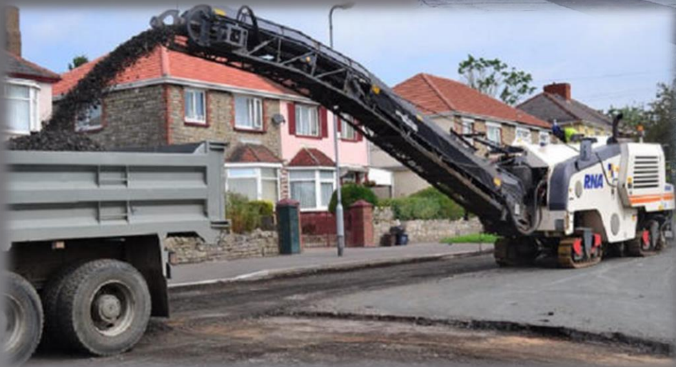
Mill and Fill Asphalt Street: $42/ft. - Contractor Mill/City Crew Fill
