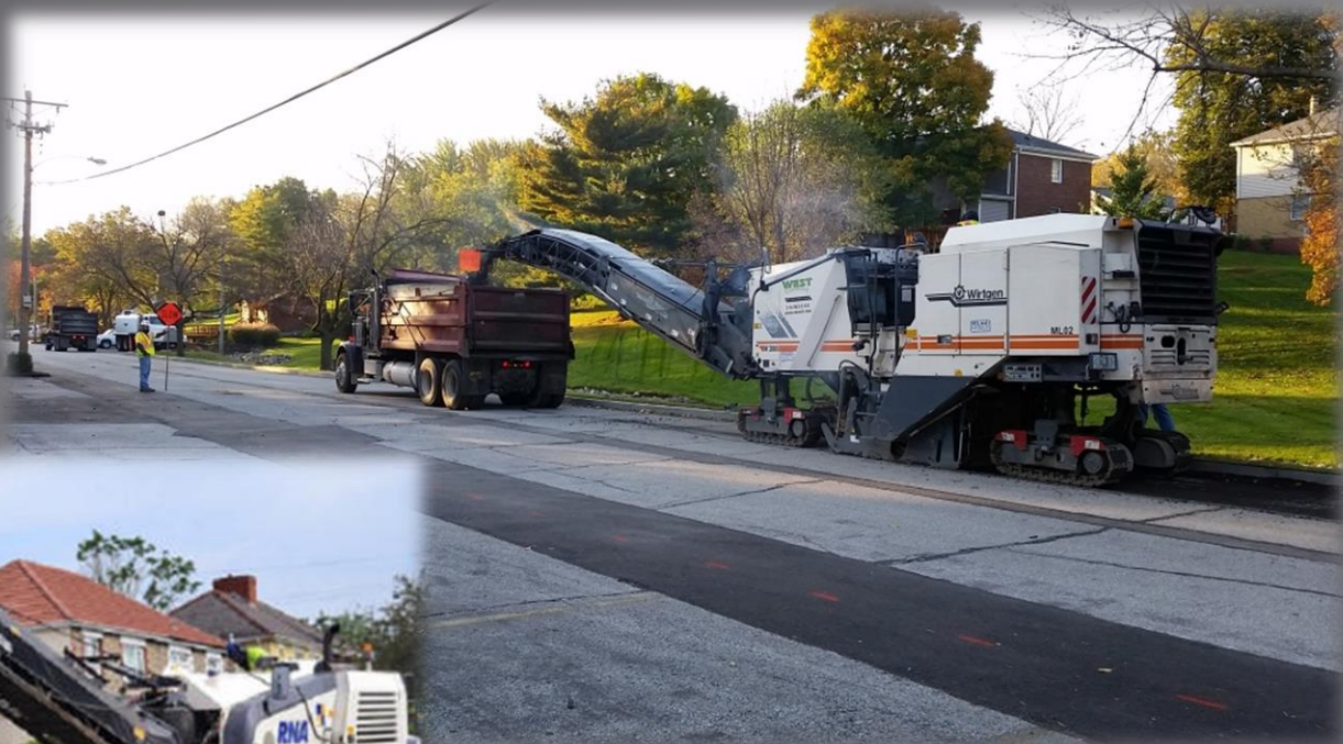
Mill and Fill Asphalt Street: $75/ft. - Contractor
