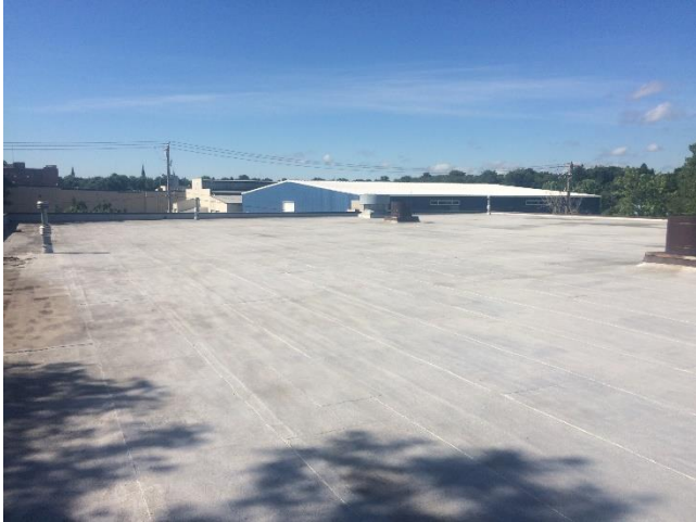
Transit Garage – Roof #3 – Overview Photo 1
