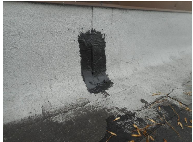
Transit Garage – Roof #2 – Open lap was repaired with 3-course of asphalt roofing mastic and fiberglass reinforcing fabric.
