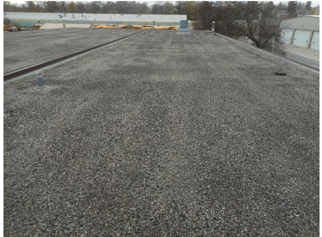
Transit Garage - Roof #4 – Overview 2
