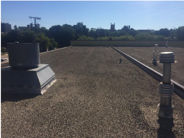
Transit Garage - Roof #4 – Overview 1
