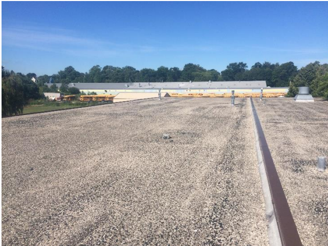
Transit Garage - Roof #5 – Overview Photo
