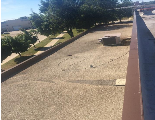
Transit Garage – Roof #1 - Overview
