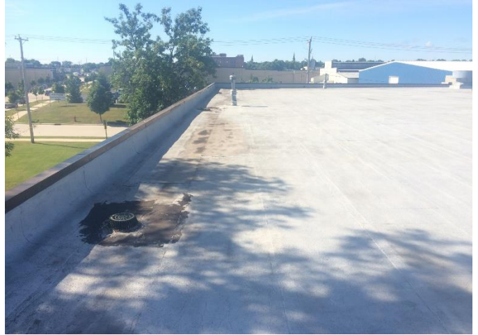
Transit Garage – Roof #3 – Overview Photo 2
