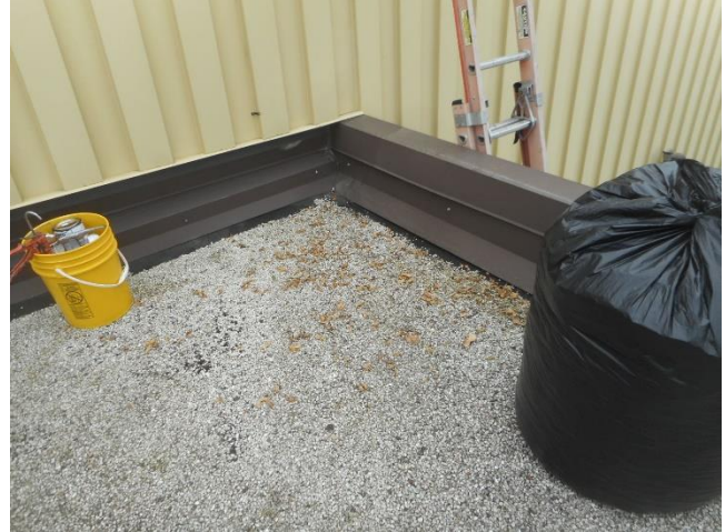
Transit Garage – Roof #1 – Debris was cleaned from roof and disposed of.
