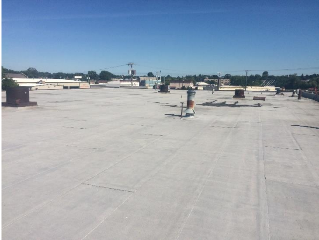
Transit Garage - Roof #2 – Overview Photo
