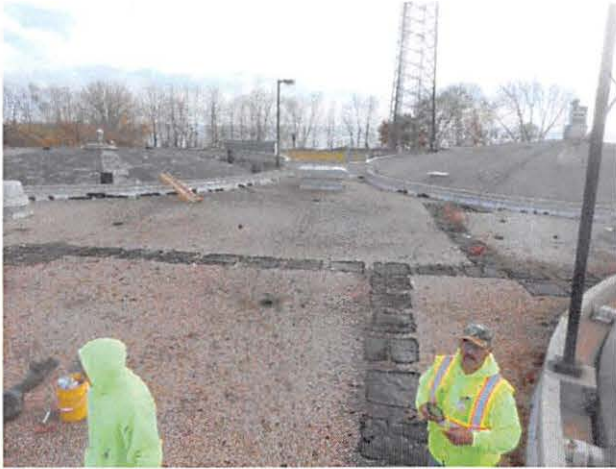
New Water Treatment Roof – Overview Photo
