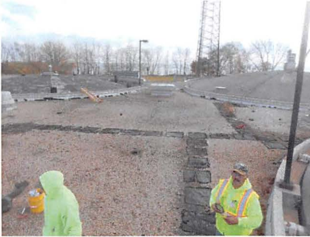
New Water Treatment Roof – Overview Photo
