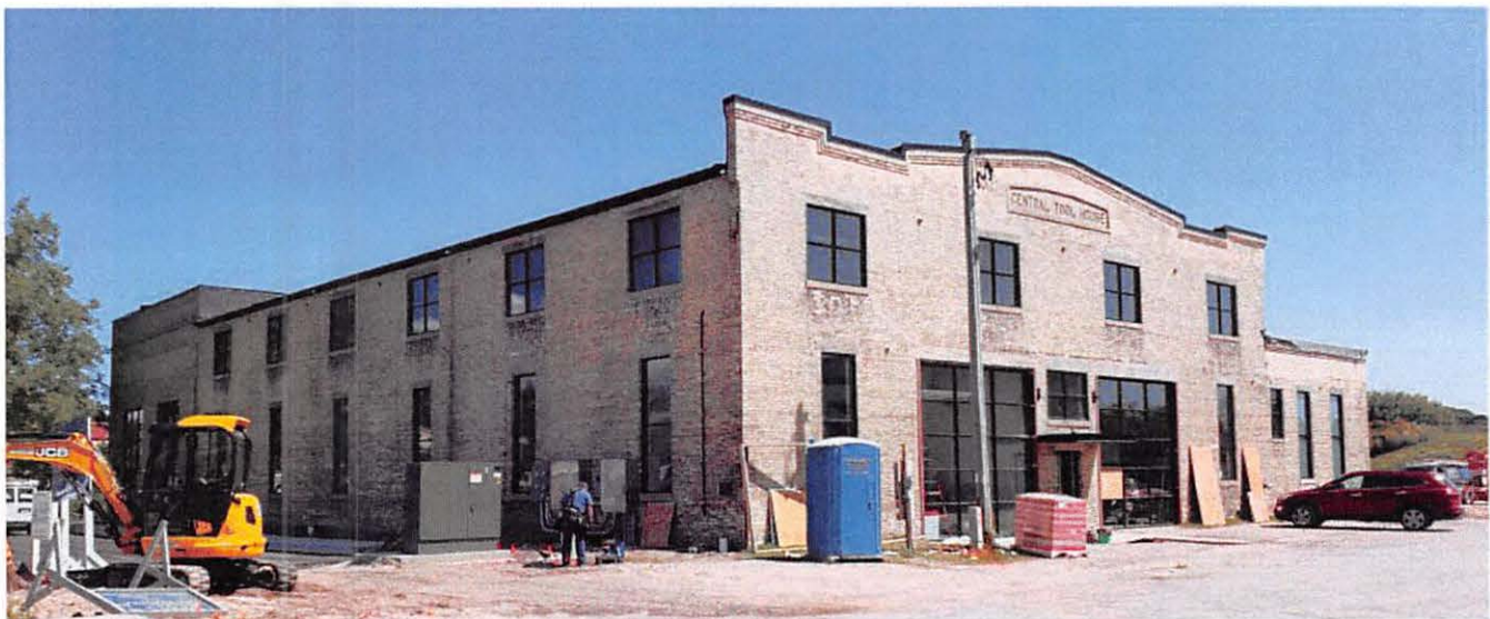
▲ A view of the ongoing historic rehabilitation efforts of 1320 Niagara Avenue. This building will feature 2-3 new mixed-use tenants.
