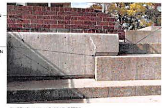
EXISTING WALL AT REAR STEPS
