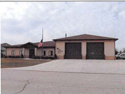
Fire Station #5 4504 South 18 th Street Ladder 5 Engine 7 (Reserve Engine)
