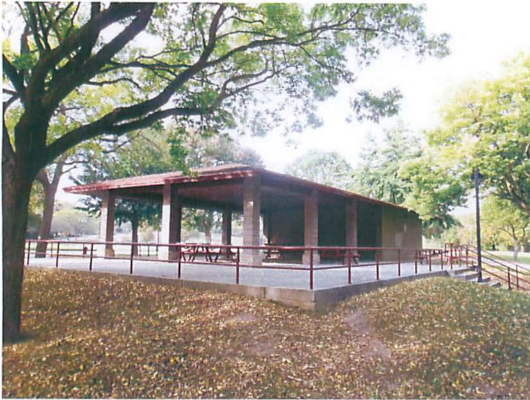
View of Main shelter looking Northwest from paved promenade
