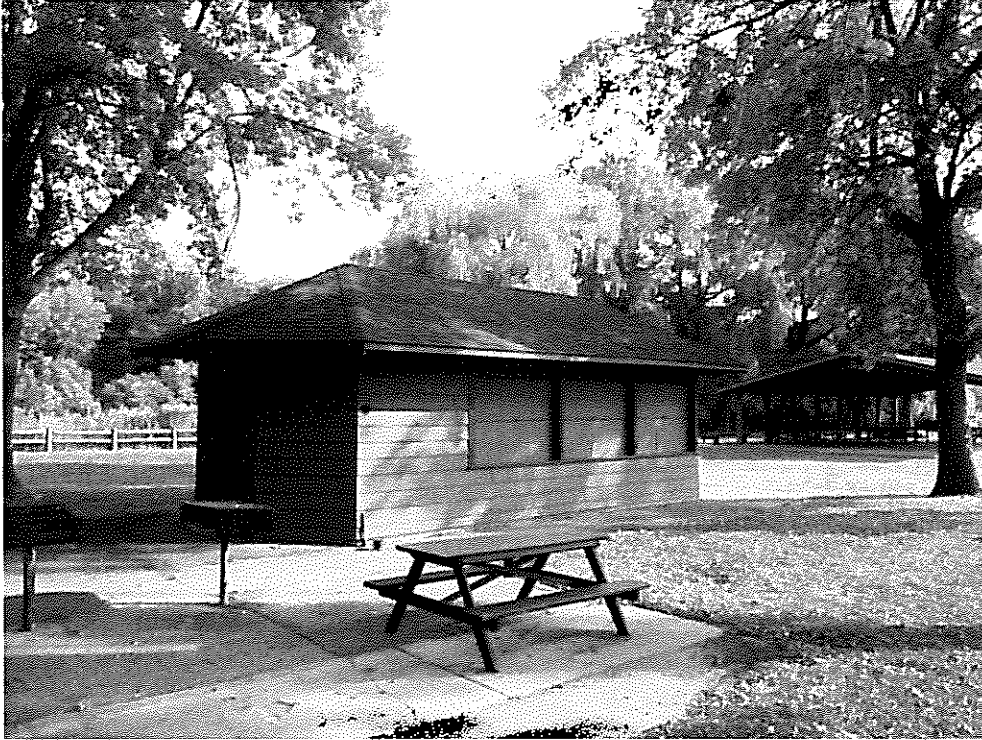
View of the concession stand from just off the patio
